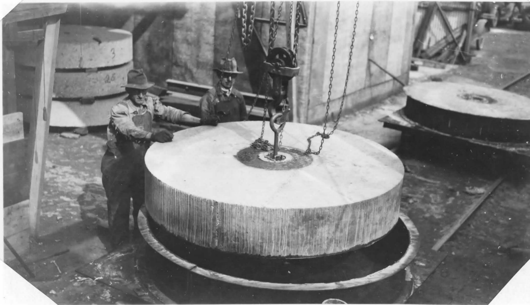
Grindstone after removal from mold. The stone is 8 feet in diameter.
