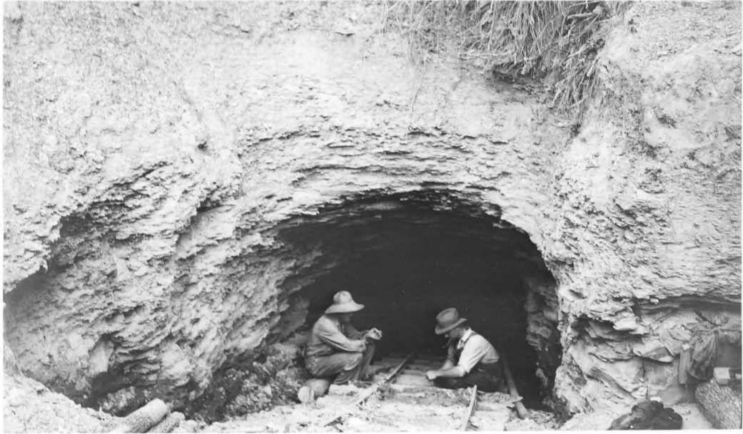
Figure 9. Entrance to Hill Mine in SE corner of Section 34, T 9S, R 4E, showing overburden of coal No. 5. The coal begins a few feet from the entrance of the mine.
