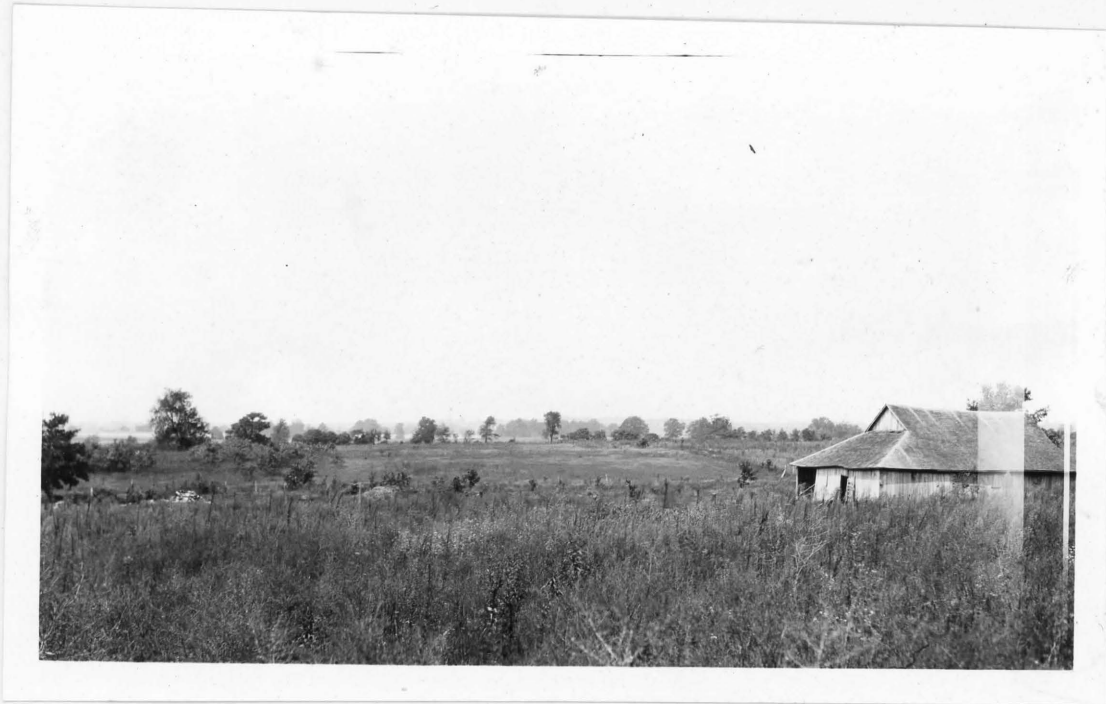
Figure 1. Surface view of East end of Carrier Mills Tract looking Southwest.
