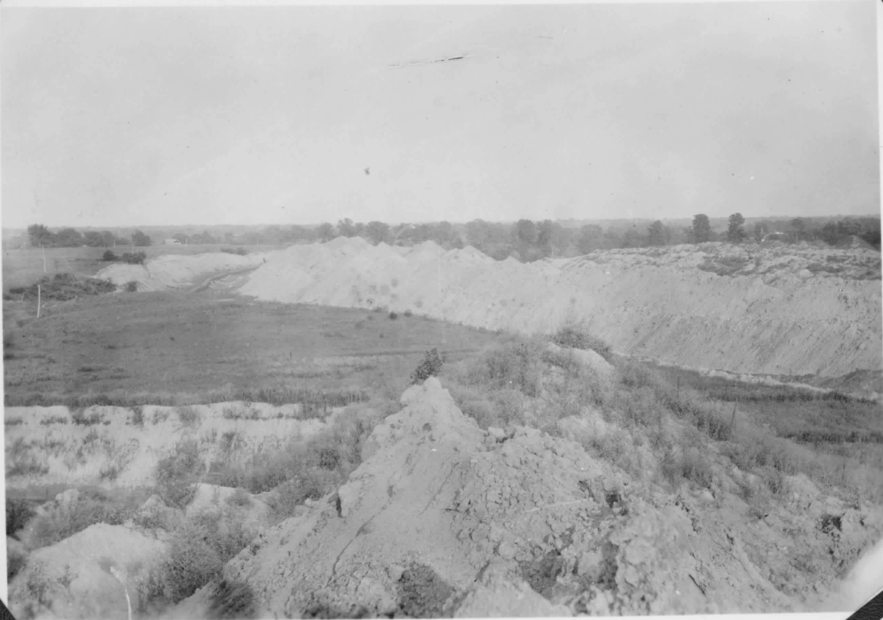
Fig. 11. PILES OF STRIP MINE DEBRIS IN THE SW. \frac{1}{4} SEC. 27, T. 6 N., R. 3 E. (Putman). wp An area from which the coal has not been removed is seen in the middle distance. The strip piles behind this area were made during 1927, the year the picture was taken. The piles in the background to the right, and in the immediate foreground were made during 1925 and 1926 and have become partially covered with vegetation.
