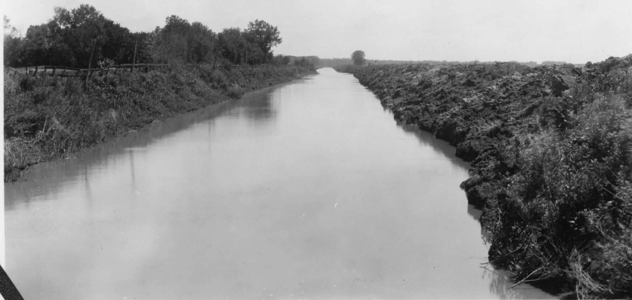
Fig. 115 . A drainage ditch and levees about three miles west of Havana. The road from Havana to ### Duncan Mills is on the levee at the left, and Spoon River is to the left of this road. A large tract of land southwest of Havana was flooded in the fall of 1926 when the waters of Spoon River broke across this road into this drainage ditch in the area shown by this picture, and the combined waters caused a break in the levee to the right, flooding all of the Langellier and Lacey drainage districts.
