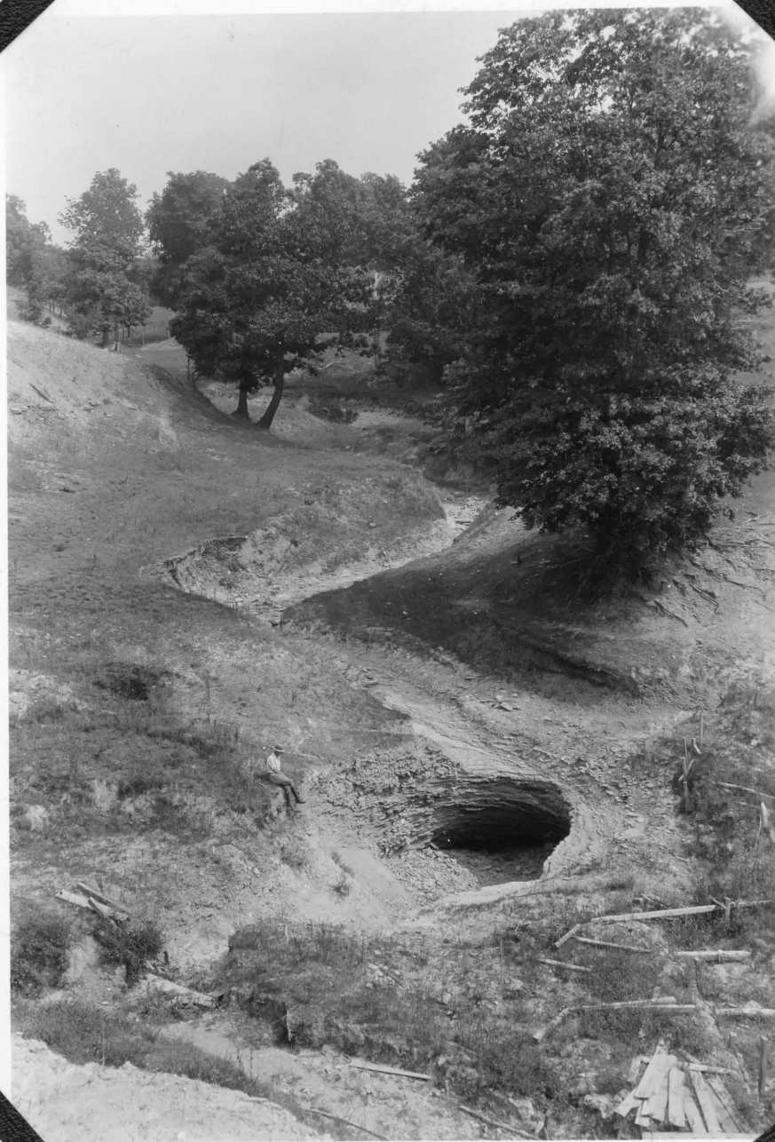
Fig. 10 . A Cave-in or sink in the bed of a ravine in the NE. \frac{1}{4} SW. \frac{1}{4} sec. 23, T. 6 N., R. 3 E. (Putman dup ), resulting from the removal of the Springfield (No. 5) coal by underground mining. This cave-in took place in July or August 1927, during the field season spent in this area. The strata exposed in the sides of the cave-in belong to the Canton Shale member of the Carbondale series. The Springfield coal is 15 to 20 feet below stream level in this locality.
