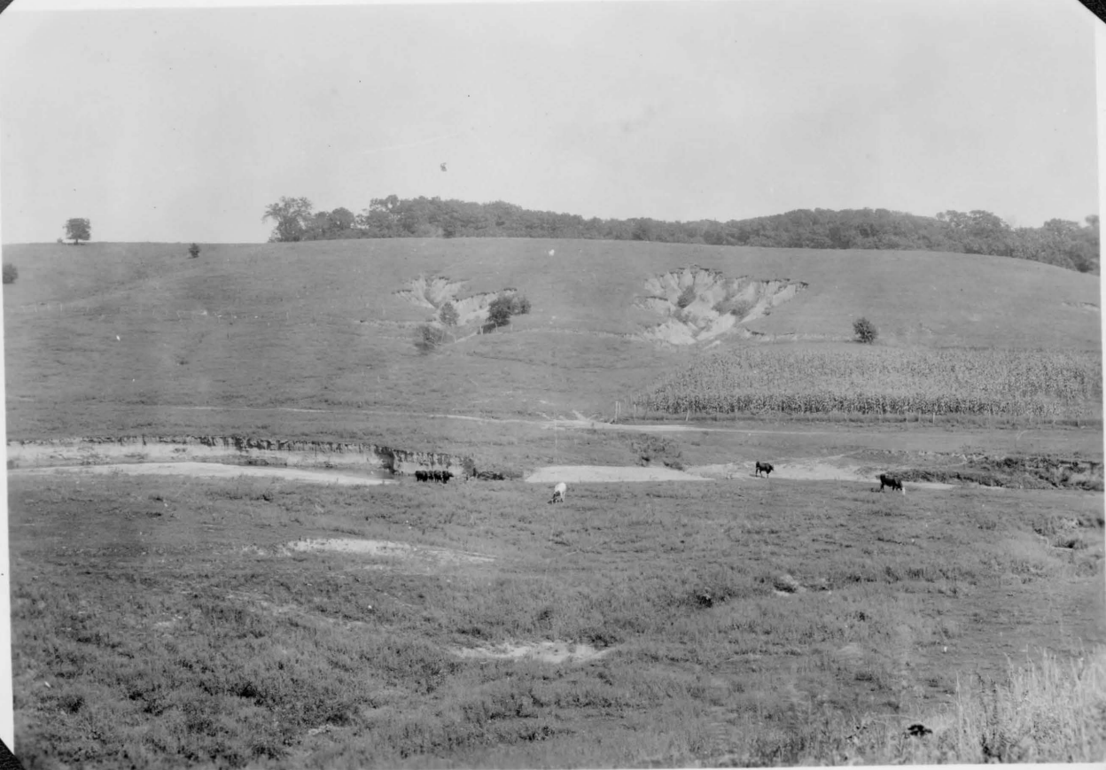
Fig. 101 . East slope of the North ### Branch of Otter Creek in the SW. \frac{1}{4} sec. 19, T. 4 N., R. 3 E. (Isabel) twp , showing the development of new systems of gullies on deforested slopes adjacent to streams. The lower slopes below the gullies are mantled with alluvial fans, ### ### composed of debris ### brought down by these gullies. These gullies are excavated in loess and Illinoian till.
