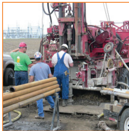
ISGS drilling and well installation at the ADM site for the monitoring, mitigation, and verification portion of the deep saline reservoir pilot program.
