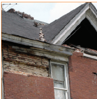
1904 Berry School, Mt. Carmel, Illinois, showing the collapsed chimney and missing bricks that resulted from the April Illinois earthquake.
