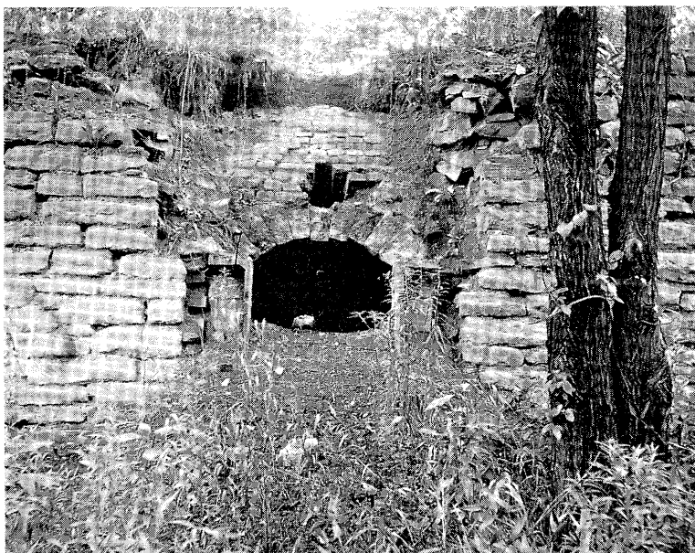
Fig. 12.—ABANDONED OVENS AT SPARTA: VIEW OF OVEN DOOR AND ARCH WITH PART OF STONE FACING REMOVED.
