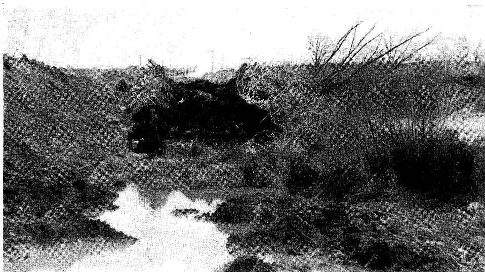
FIG. 23.—Muck and peat heaved by a highway fill across a swamp along 104th Avenue (Flavin Road) just south of 95th Street.
