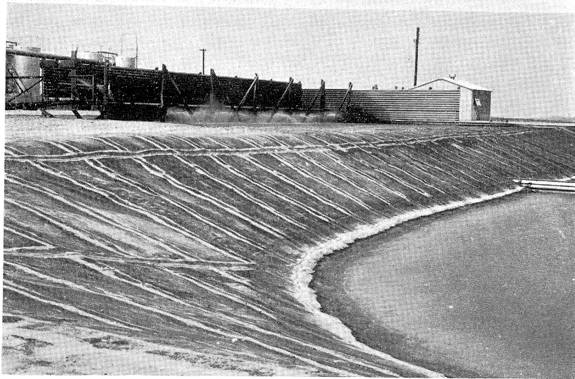
FIG. 8 (Above).—Mixing and flocculation basin, showing arrangement of “end-around” baffles.
