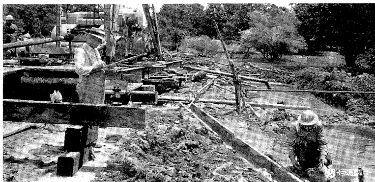
"Catching samples" of drill cuttings at a well for study of possible producing reservoirs.
