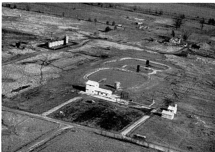
Figure 3—The Water Plant at the Patoka Water Flood Operation. The water well pumps from the Tar Springs formation. The salt water is aerated above the most distant pond, and settled there. It is treated in an accelerator and filtered in the largest of the buildings. The water is distributed by centrifugal pumps to the water input wells throughout the field.
