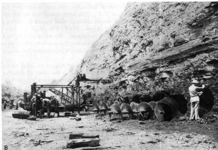
A. - Strip mining Davis and DeKoven coals, Stonefort Township, Saline County. B. - Open-cut and auger mining the No. 5 coal, south limb of Eagle Valley syncline near Lemington, Gallatin County.
