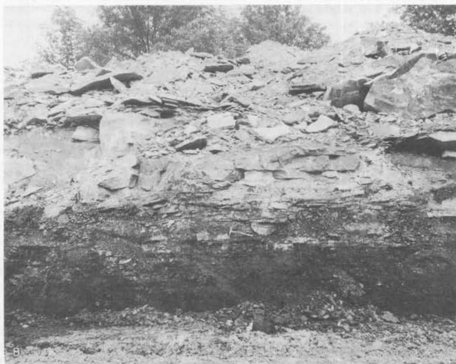
A. - Strip mining the New Burnside coal near New Burnside, Johnson County.
