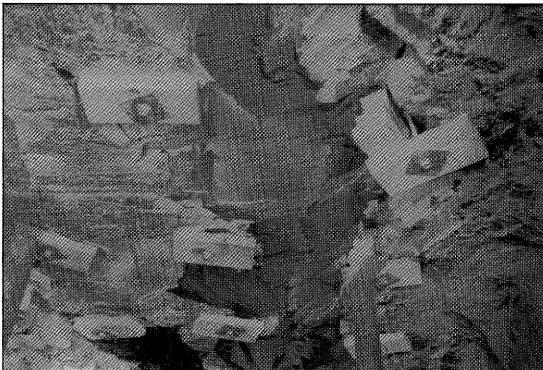
Figure 26 "Kink zone" caused by horizontal stress in mine roof.
