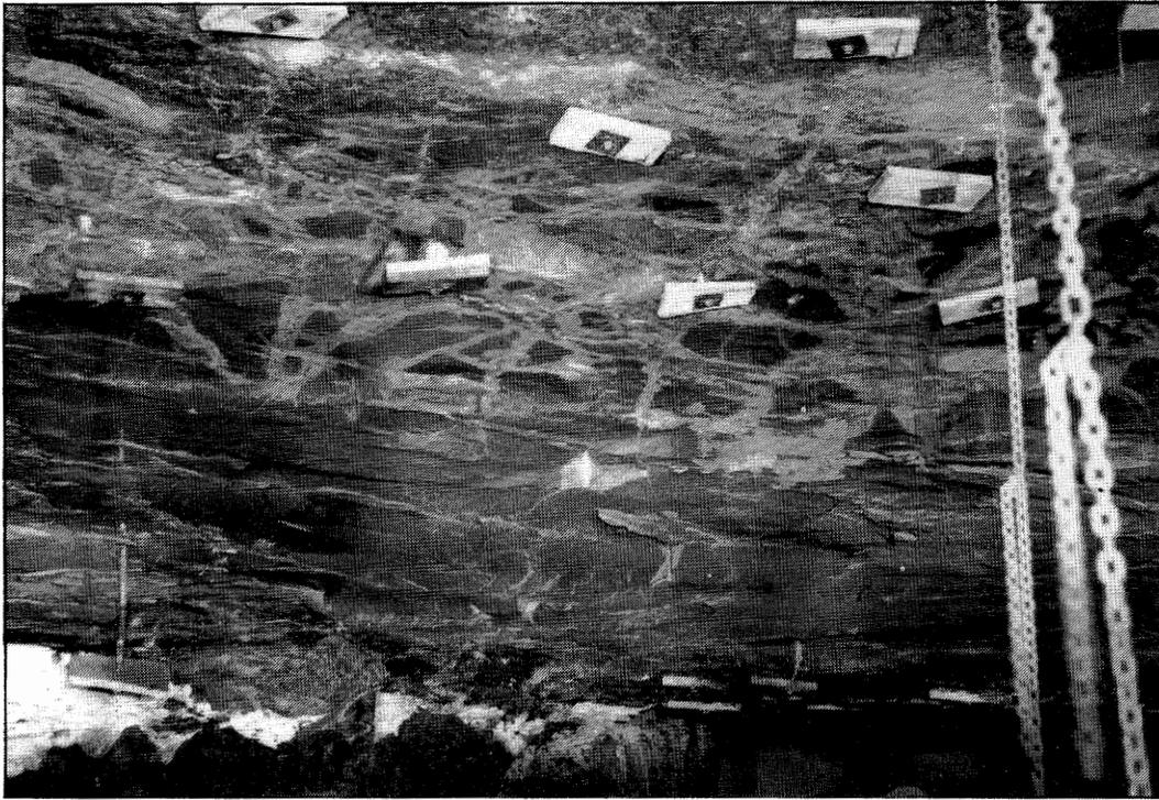
**Figure 14** Lawson Shale here is immediate roof. Lower part is dark and massive; upper part is mottled and penetrated by light-colored syneresis cracks. This shale is difficult to support in mine roof.
