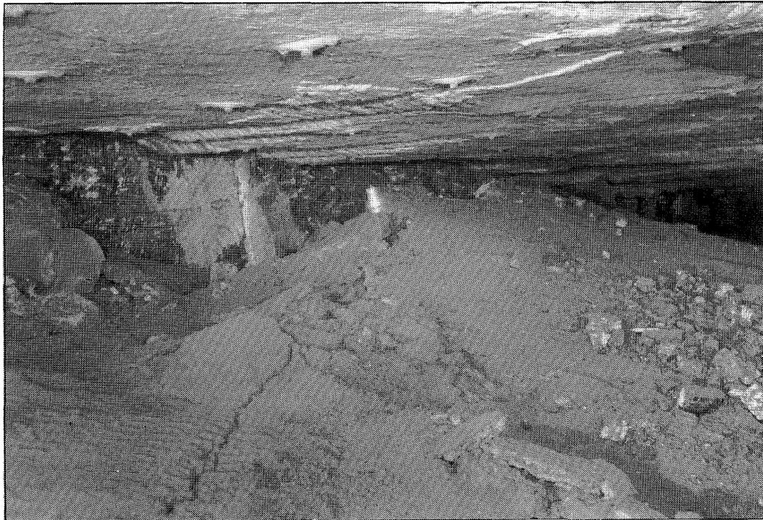
**Figure 24** A severe floor heave or squeeze occurred here; pressure on pillars forced plastic underclay into mine openings. In this example the roof remains intact.
