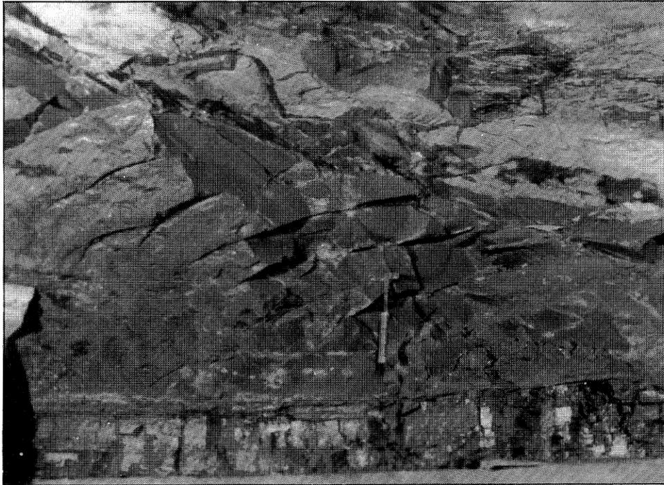
**Figure 7** Edge of a lens of Energy Shale, overlain by Anna Shale (upper right). Numerous slip-fractures make Energy Shale difficult to support. Photo from Spotti (1941).
