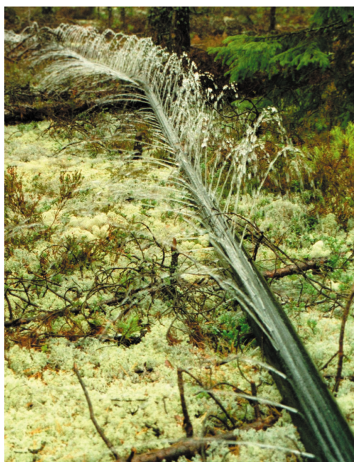
Figure 2 Artificial recharge by the sprinkling method. (Photo courtesy of J. Kääriä, Turku Region Water Ltd.)
