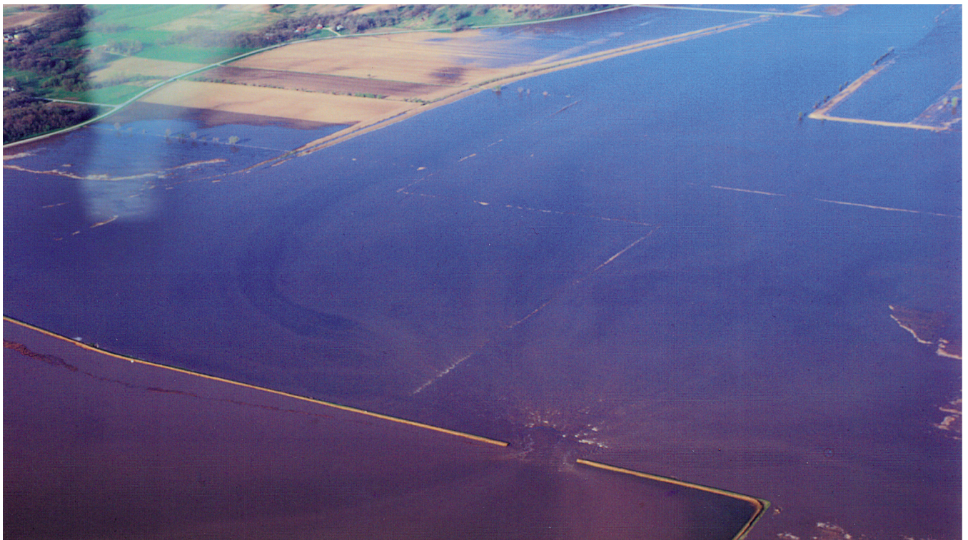
Figure 22 Breach in the Little Meredosia Levee. This view to the southwest was taken April 4, 1973.
