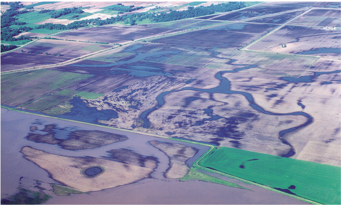
Figure 23 Repaired Little Meredosia Levee during the 1974 Rock River flood. This view to the southwest was photographed May 24, 1974.
