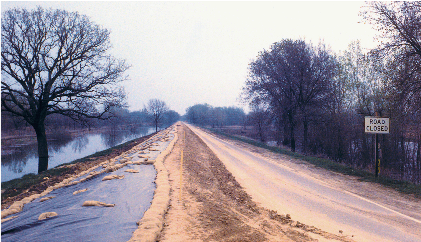
Figure 19 Temporary levee built on Illinois Route 84 to protect the flooded Meredosia Channel, on the right, from Mississippi River floodwaters, on the left. The photograph was taken April 4, 1969.
