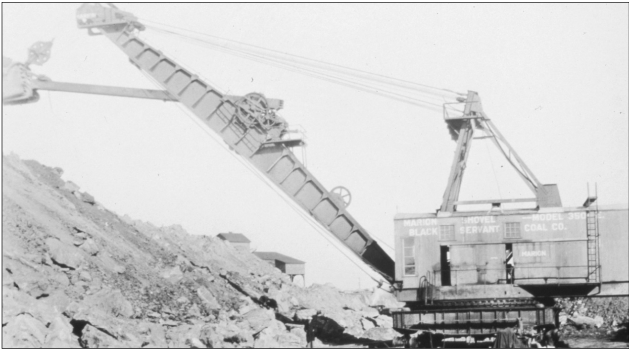
Figure 192 Black Servant Coal Company, Jackson County. The Marion 350E had an 8-cubic yard bucket and a 90-foot boom, weighing in at 560 tons (Historical Construction Equipment Association 2002). The shovel shown is rail-mounted, but this model was the first that Marion fitted with crawlers (Bottomley 1944).
