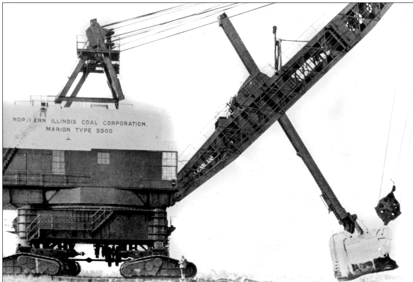
Figure 199 Northern Illinois Coal Corporation, near Wilmington, Will County. The Marion 5560 shovel, with a man standing next to it for scale, had a 32-cubic yard bucket (Sheley 1935). During the 1930s, steel alloys and aluminum were used, and the dippers were welded rather than cast, which made them lighter and stronger.
