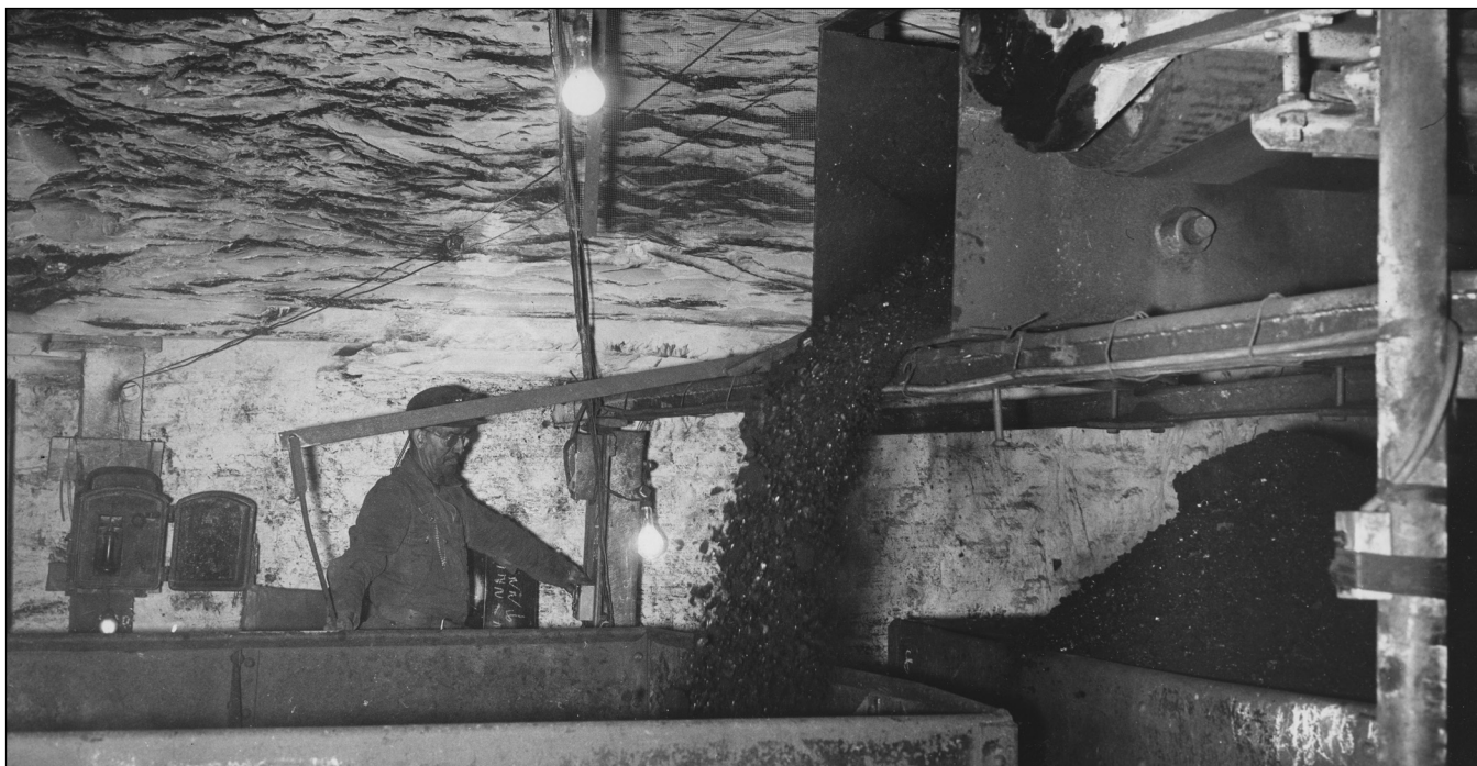
Figure 77 Sahara Coal Company, No. 5 Mine, Saline County. Coal is transferred from a rubber panel belt to coal cars for haulage to the shaft bottom, a hybrid system used before belt haulage totally replaced track haulage. A moveable baffle prevents coal spillage between cars (Ledvina et al. 1992).
