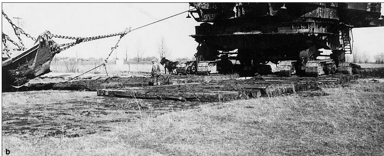
Figure 204 Northern Illinois Coal Corporation, Northern Mine, Will County. The Marion 5480 dragline, weighing about 975 tons (Historical Construction Equipment Association 2002), could carry and lay down timbers to protect the roads and fields from the compression of this enormous weight. The timbers would distribute the weight to a larger area than the crawlers that supported the machine.
