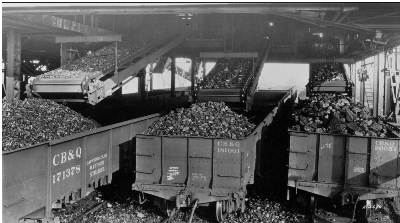
Figure 125 Mine and location unknown. The end product of the sorting process was clean coal of uniform sizes. Each size had a different market (Ledvina et al. 1992).
