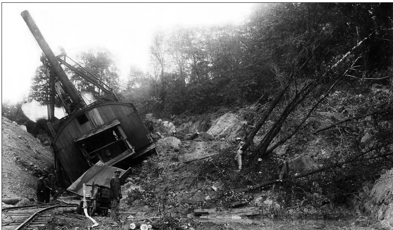
Figure 187 Mine and location unknown. Slope stability of the highwall is an important factor in surface mining. In this instance, the highwall has slumped, and the small resulting landslide has pushed the steam shovel against the spoil pile.
