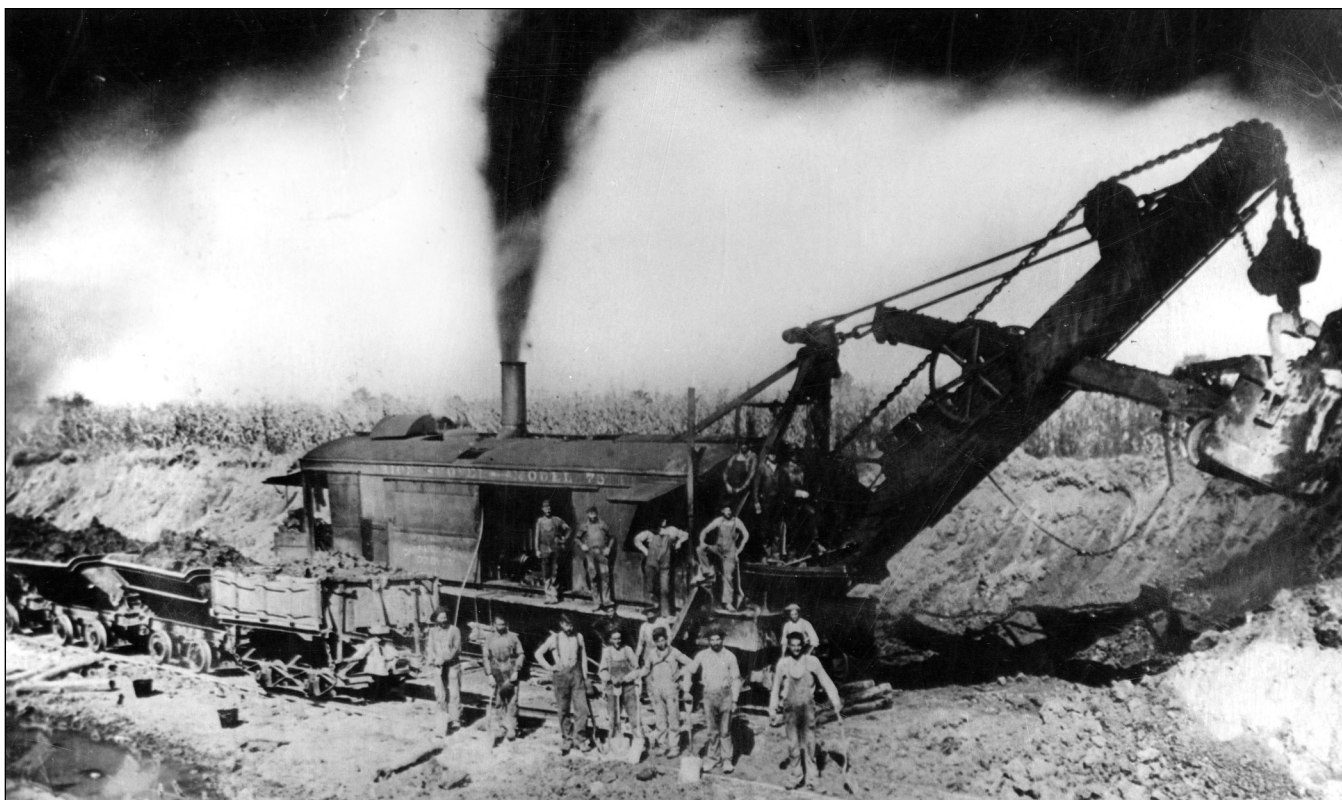
Figure 174 Fairmount Quarry, Vermilion County. This Marion Model 73 steam shovel is working in a gravel pit. The chain that controls the bucket, the short massive boom and dipper stick, and the 180-degree rotation allowed on the rail-mounted foundation are similar to the earliest coal mining steam shovels in use since 1877. A steam-powered locomotive is probably just out of the picture on the left (indicated by the vast amount of black smoke in that portion of the picture). The pit cars are emptied by tipping them to the side. The end car has a hoist mechanism to aid the process. The size and strength of pit cars increased to keep pace with shovel developments so that the same number of cars were kept occupied (Phelps 1973).
