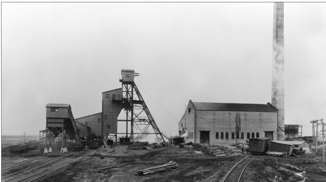
Figure 5 Old Ben Coal Corporation, No. 11 (or New North) Mine, Franklin County. Mines often constructed railroad spurs that stored the cars for hauling their coal to market. The large A-frame structure (head frame) in the center was the location of the hoist shaft, and the building to the left was the sorting shed and tippie. A pile of timbers to prop the mine roof can be seen in front of the building on the right, which probably contained mine offices, hoisting equipment, and machine shops. This mine was the site of an explosion on Thanksgiving Day in 1917.
