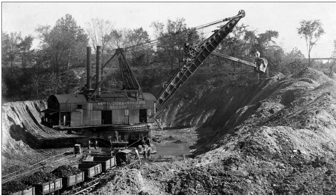
Figure 181 Mission Mining Company, west of Danville, Vermilion County. This Marion 300 steam shovel had a 6-cubic yard bucket and weighed 350 tons (Historical Construction Equipment Association 2002).
