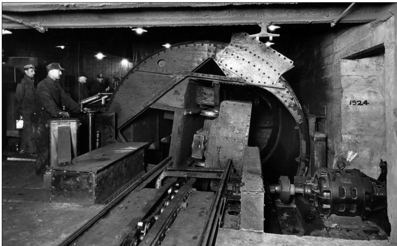
Figure 108 Chicago, Wilmington & Franklin Coal Company, Orient No. 2 Mine, Franklin County. Rotary car dump. In mines of this vintage, cars were often hoisted directly and dumped on top. In this mine, a rotary dumper emptied the cars into a bin, and the coal was then hoisted by “skips”—large open cars or buckets (Ledvina et al. 1992).
