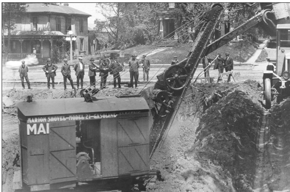
Figure 185 Digging for the foundation of the Harding Hotel in Marion, Ohio. The Marion 21 shovel had a \frac{3}{4} -cubic yard bucket that was very popular and was offered with steam, gasoline, or electric power. More than 800 were sold between 1919 and 1927 (Historical Construction Equipment Association 2002). These shovels were likely used in Illinois coal mines for loading coal.
