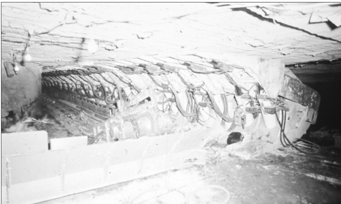
Figure 102 Old Ben Coal Corporation, mine and location unknown. This end of the longwall face shows the side of the shield supports.
