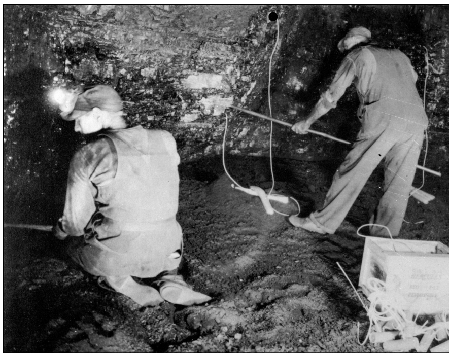
Figure 42 Muddy Valley Mining Company, Hallidayboro Mine, Jackson County. When coal was shot with black powder or permissible explosives, the charge had to be primed and tamped into place, and the wires or fuse carefully routed out the hole collar. The end of the hole was then stemmed with some inert material (Ledvina et al. 1992). The box is labeled “Hercules permissible” explosives.
