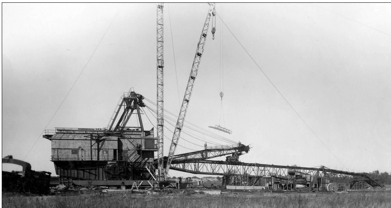
Figure 215 Fairview Collieries Corporation, Harmattan Mine, Vermilion County. The final stage of construction is to attach the boom and the bucket to the boom. Steel towers with wire rope guide lines are erected to enable raising the boom to its position against the dragline housing. To show the scale of the machine, a man is barely visible standing on the upper gantry of the boom.
