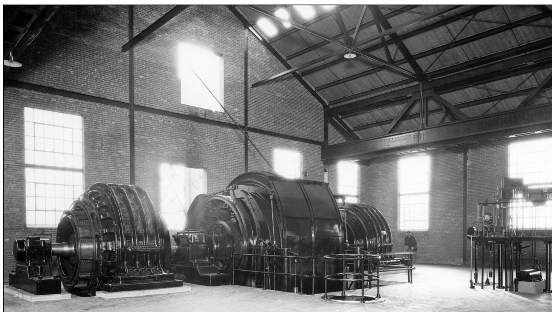
Figure 116 Bell & Zoller Coal Company, No. 1 Mine, near Zeigler, Franklin County. This dual-cylinder hoist operated the twin cages hauling coal cars in the 400-foot-deep shaft. These early steam hoists generally outperformed their modern electric counterparts (Ledvina et al. 1992). The man operating the engines is the hoisting engineer, who was in charge of raising and lowering the cage. The headframe is visible through the gap in the wall in front of the engineer. The headframe is the housing for the cable that raises and lowers the shaft mechanism, controlled at the surface.
