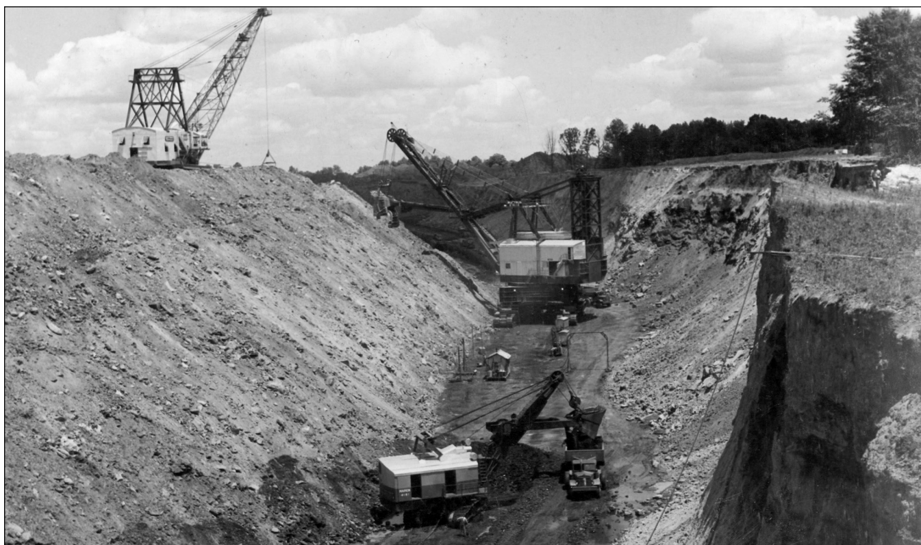
Figure 223 Mine unknown, perhaps Harmattan Mine, Vermilion County. This photograph shows the typical configuration of surface mines in the latter half of the twentieth century. The dragline on the spoil pile rehandled the spoil so that the piles did not slide back into the pit as the shovel added material. A bulldozer cleaned the top of the coal and sometimes aided the loading shovel.
