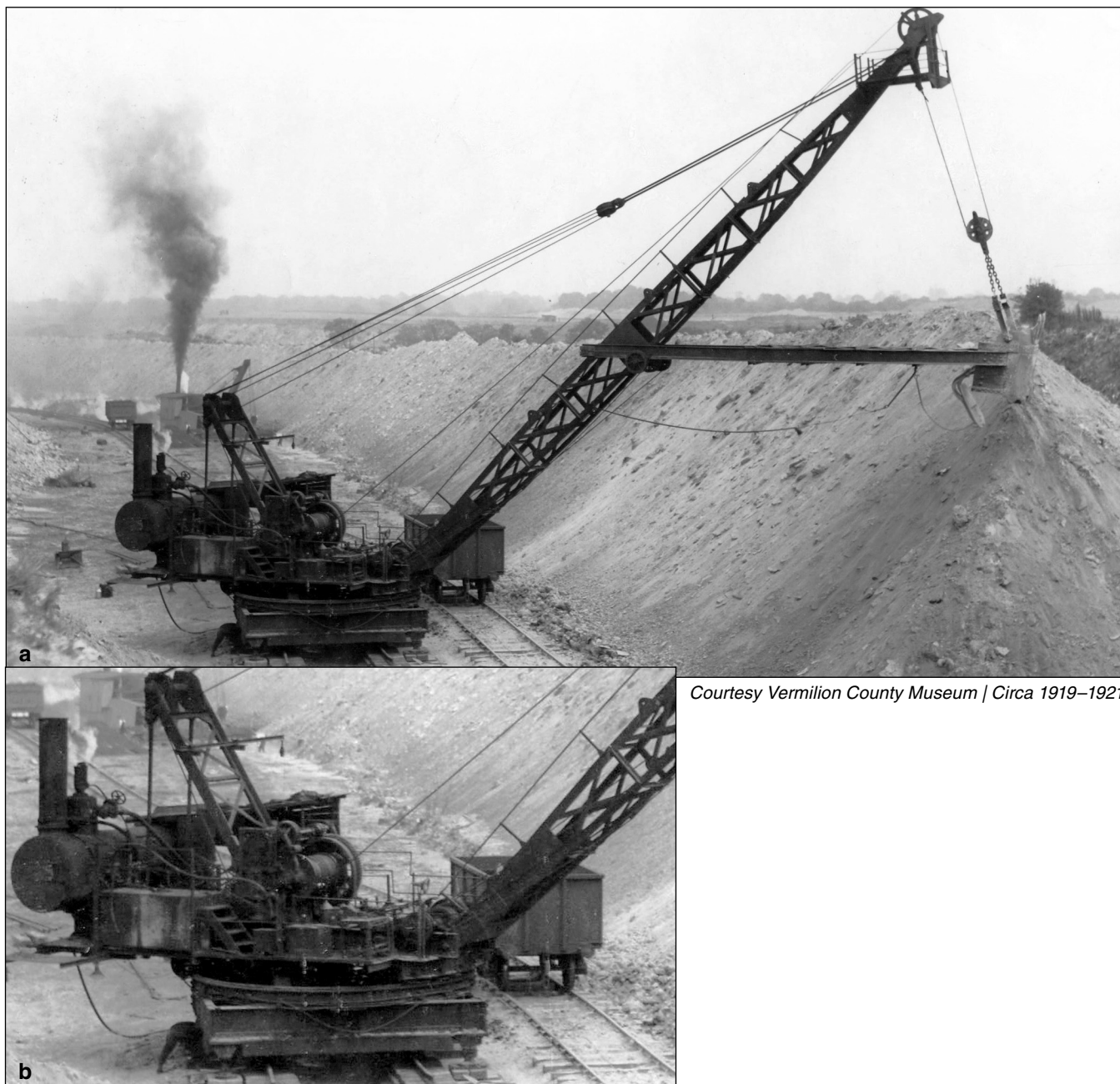
Figure 184 Location unknown, probably in Vermilion County. (a) This photograph is a rare shot of a steam shovel without a housing so that all the works are visible. The steam tank was in a horizontal configuration; these tanks generally were vertical. The shovel was supported on hydraulic jacks to keep the machine level, and the shovel revolved fully to remove overburden (left side of the photograph) and deposit it (right side of the photograph). Shovels increased about fourfold in size between 1912 and 1927 (Williamson and Myers 1955). Equalizing devices were incorporated into design modifications to enable the huge excavators to operate on uneven surfaces. Marion Shovel Company used hydraulic jacks at the corners of the undercarriage, whereas Bucyrus Company's solution was a patented equalizing beam that provided three-point suspension (Williamson and Myers 1955). (b) Enlargement of the suspension and steam tank of the steam shovel.
