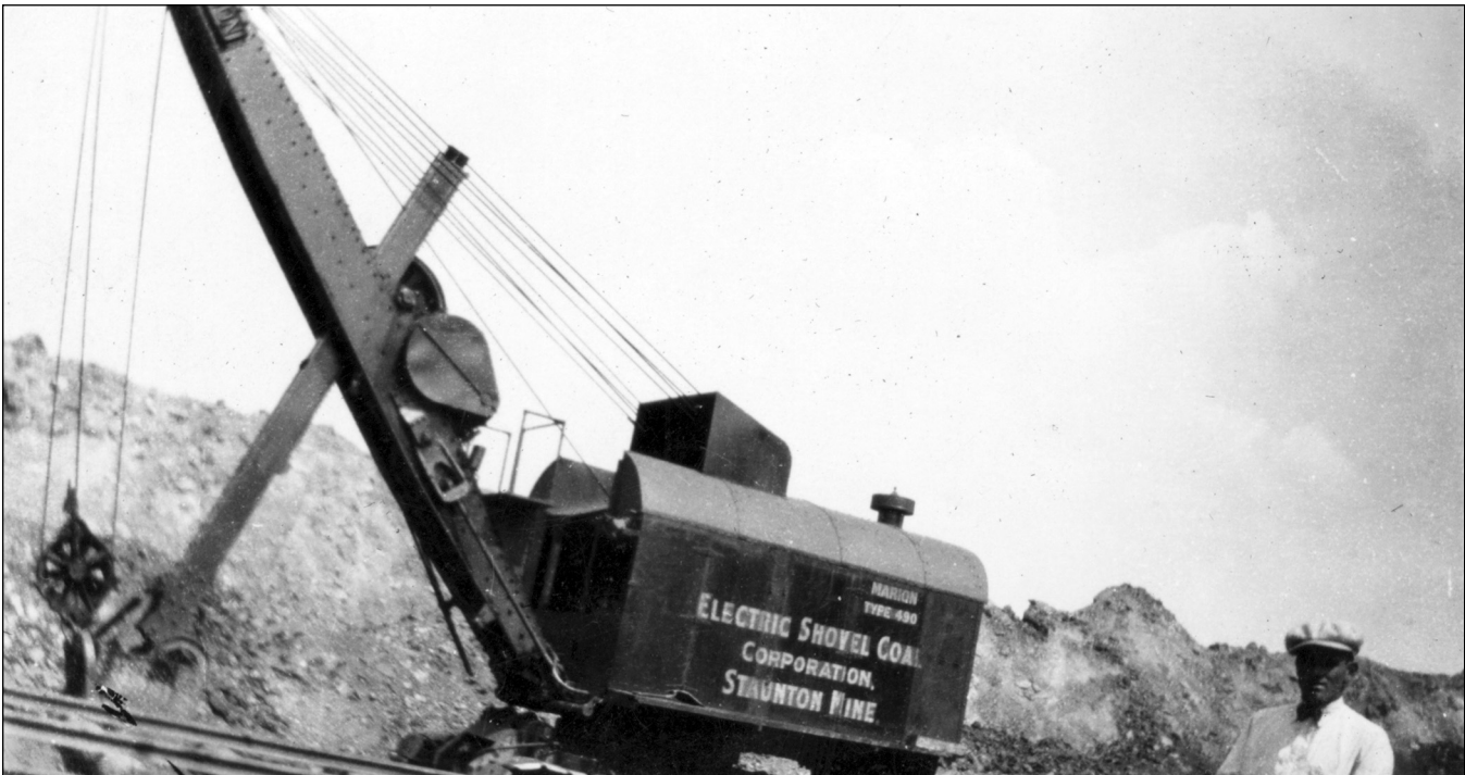
Figure 193 Electric Shovel Coal Corporation, Staunton Mine, Vermilion County. A Marion Type 490 shovel with a 2¼-cubic yard bucket (Historical Construction Equipment Association 2002) is shown on crawlers. The underframe of the shovels had to be reinforced to mount them because less attention was given to the preparation of the roadway for a crawler-mounted shovel. The design for the underframe was made more rigid to compensate for the unequal weight distribution, and the depth of the underframe was increased (Sherwood 1943).
