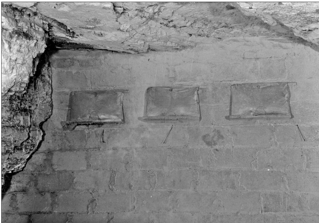
Figure 161 Old Ben Coal Corporation, mine unknown, Franklin County. These concrete blocks make a permanent seal for abandoned parts of an underground mine. The bags containing rock dust are designed to rupture if the seal is blown out by an explosion.
