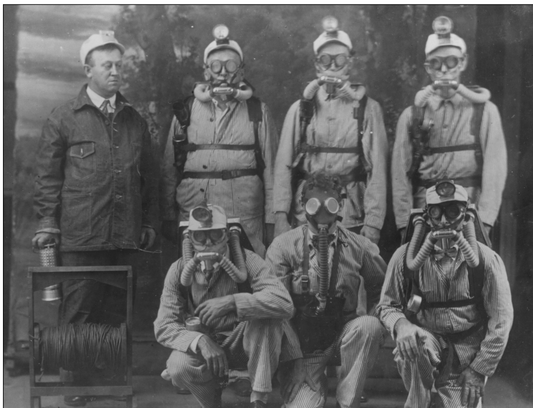
Figure 166 Madison Coal Corporation, No. 9 Mine, Williamson County. The rescue team is shown wearing rescue gear. The boxes were carried on the backs of rescuers and probably filtered carbon dioxide and carbon monoxide out of smoky air. The man in the center of the front row is the only one with gear that would have allowed him to breathe in a gassy mine. The electric cap lights of this time were very poor and produced only two-candle power or less of illumination (Jones 1954). The man on the left in the back row is holding the safety lamp.
