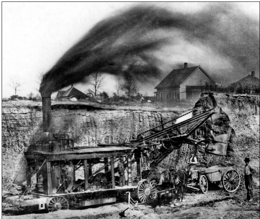
Figure 172 Mine unknown, Missionfield District, Vermilion County. A very early steam shovel removing overburden.
