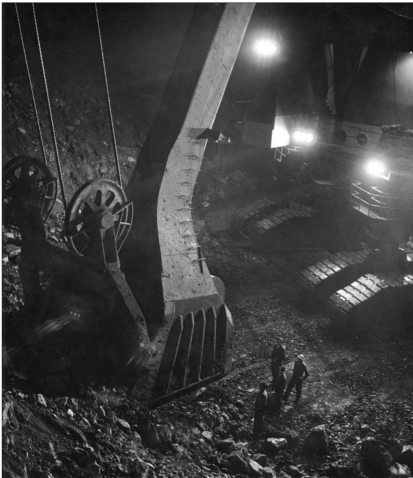
Figure 237 Peabody Energy, mine and location unknown. Coal mines often work 24 hours a day, 7 days a week. Surface mines are no exception. This photograph also shows the brackets used for handholds and footholds for maintenance on the bucket or dipper stick.
