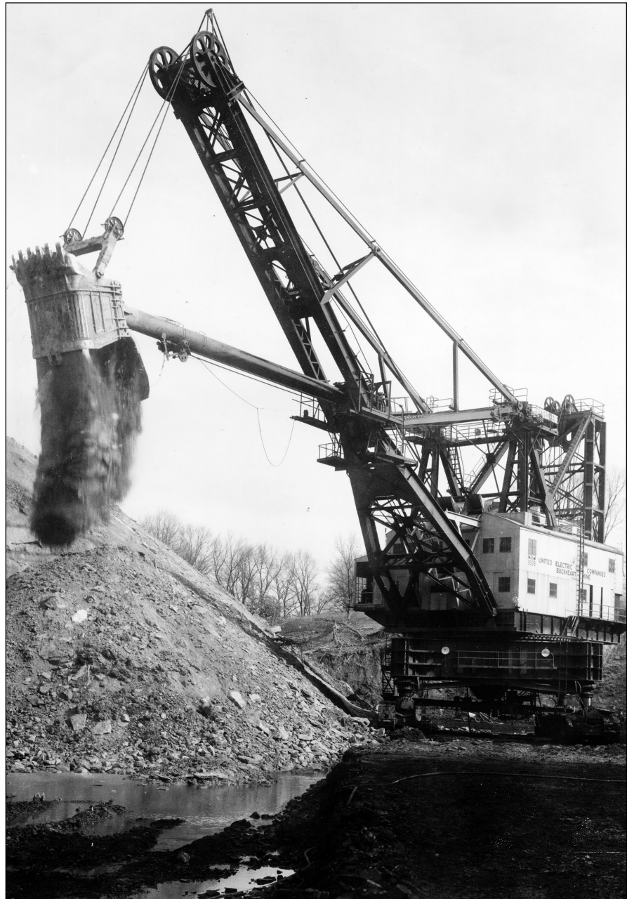
Figure 207 United Electric Coal Company, Buckheart Mine, Fulton County. The Bucyrus-Erie 950-B was a workhorse shovel that was included in many mine plans.
