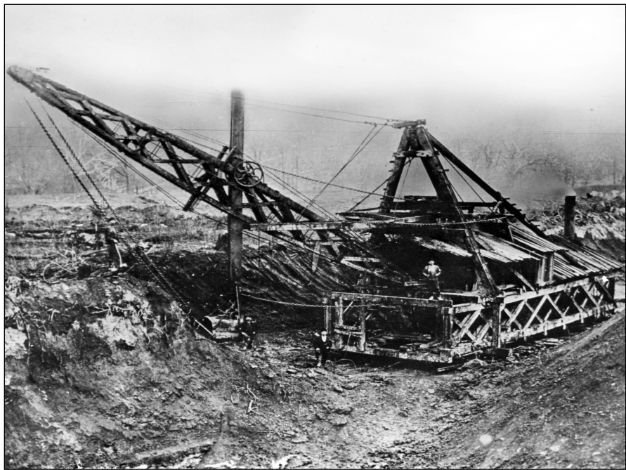
Figure 171 Missionfield Mine, west of Danville, Vermilion County. This very early stripping shovel was steam-powered. The wooden frame supports dredge machinery, making what is essentially a dry-land dredge.
