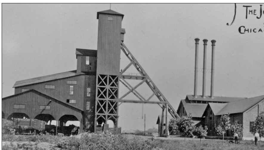
Figure 4 Springfield Colliery Company, Sangamon County. The A-frame structure in the center of the photograph is the headframe, supporting cables from the engine house on the right. The shaft is below the tower. The structure on the left is the tippie, or loading platform, and the sorting shed is above the tippie.
