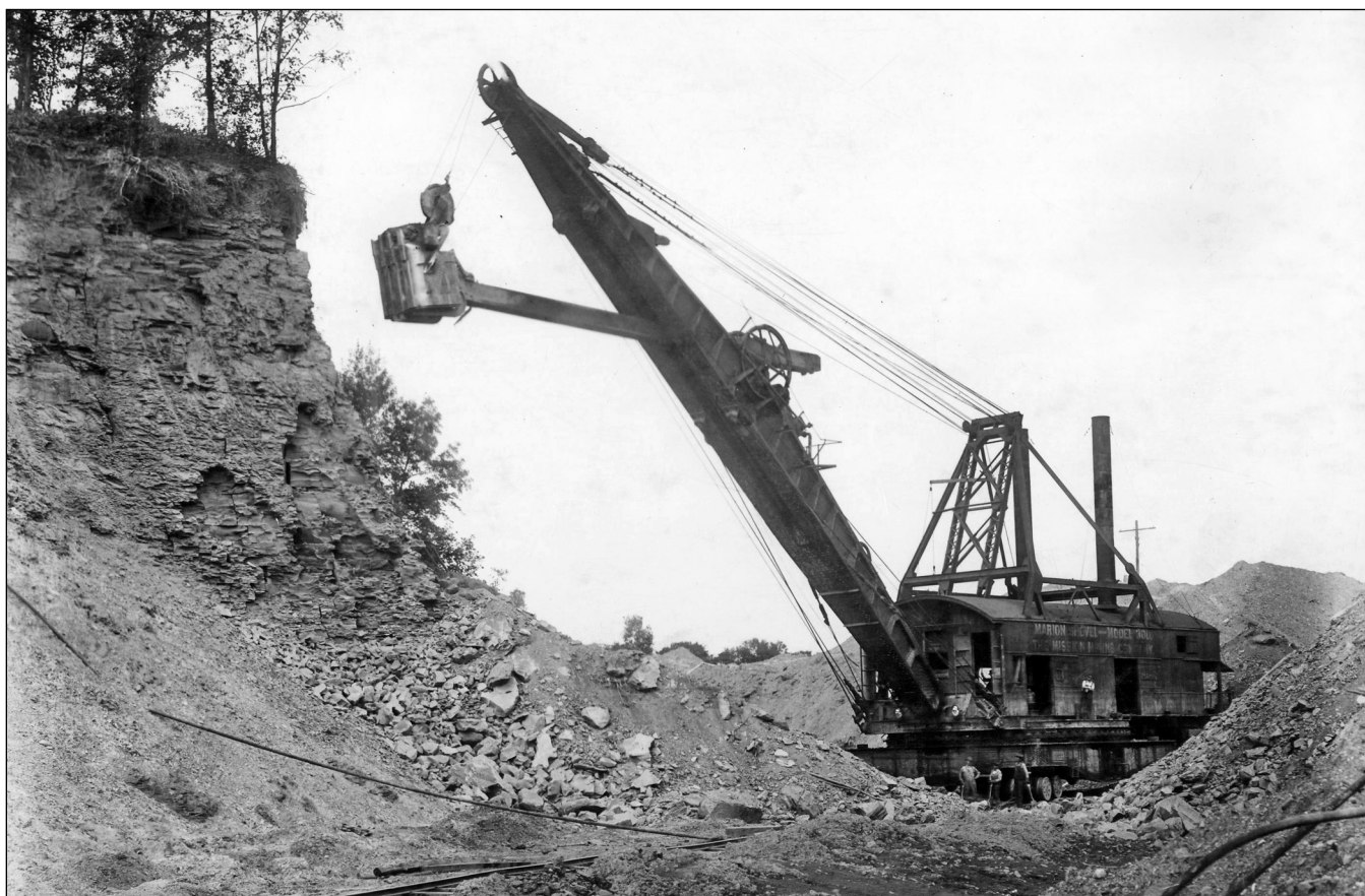
Figure 186 Mission Mining Company, west of Danville, Vermilion County. This Marion 300 steam shovel shows the depth of overburden that could be removed with these new large shovels.
