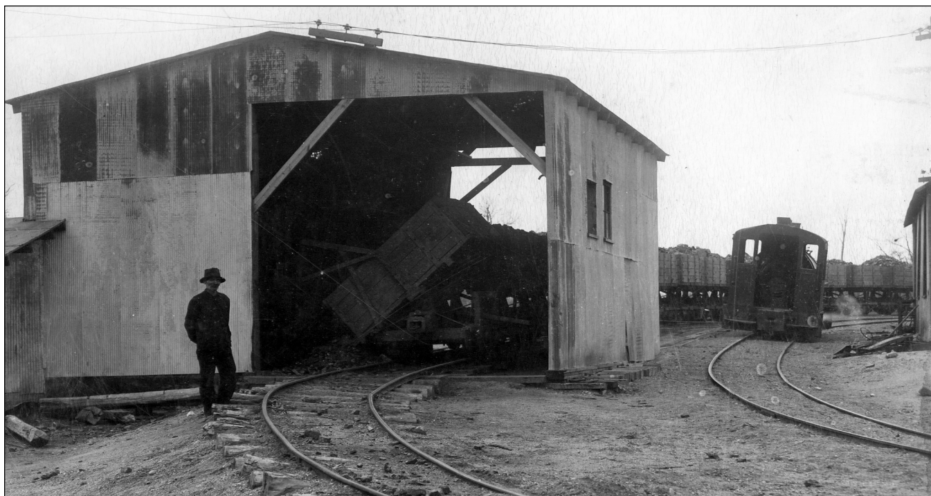
Figure 190 Mine and location unknown, probably Vermilion County. At this mine, the coal cars were emptied inside a shed. These cars had a mechanism underneath that hoisted one side of the car to dump out of the opposite side.
