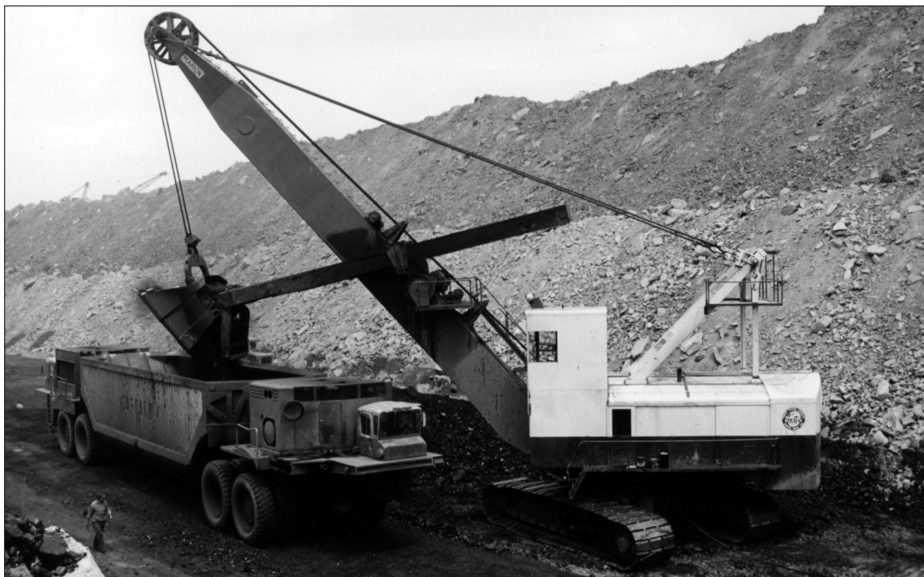
Figure 232 Southwestern Illinois Coal Corporation, Captain Mine, near Willisville, Perry County. This 240-cubic yard truck is being filled by a Marion loading shovel. Cabs in both front and back of the truck mean that the awkward vehicle does not have to be turned around, which could save considerable time in the confines of a narrow pit or loading facility.
