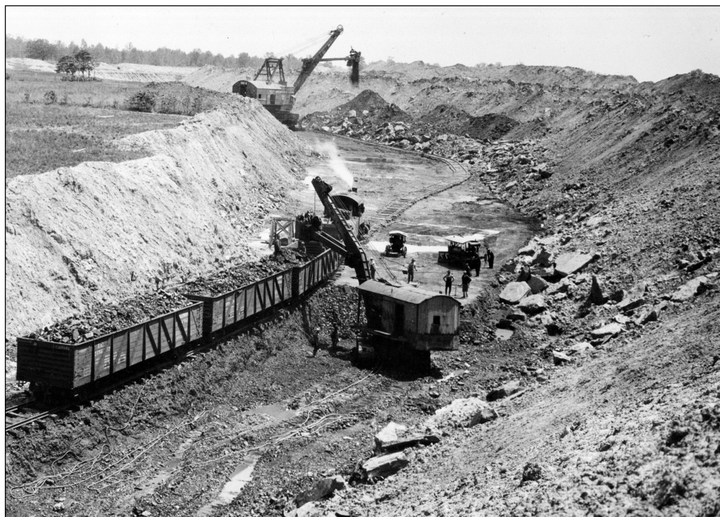
Figure 212 United Electric Coal Company, Cuba Mine, Fulton County. This is the first wheel excavator, pioneered by Frank F. Kolbe of United Electric Coal Company. Kolbe wanted an economical method of moving a great volume of soil and shale and depositing it far enough away to prevent the spoil pile from sliding back into the pit (Hollingsworth 1963). This wheel excavator could deposit to a spoil pile 400 feet away. Bucyrus built the upper portion, which was attached to a Marion dragline base. The machine weighed about 1,000 tons and had an output of 1,000 cubic yards of material per hour. This volume is about five times that of the Marion dragline model that the base was taken from (United Electric Coal Companies 1949).
