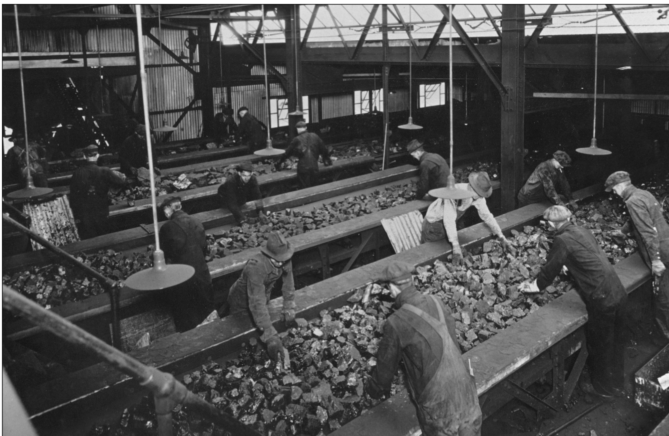
Figure 122 Chicago, Wilmington & Franklin Coal Company, Orient No. 2 Mine, near West Frankfort, Franklin County. Picking tables show the intermediate stage between grinding and loading coal into rail cars. Nothing topped hand-picking for removing roof shale from lump coal (Ledvina et al. 1992).
