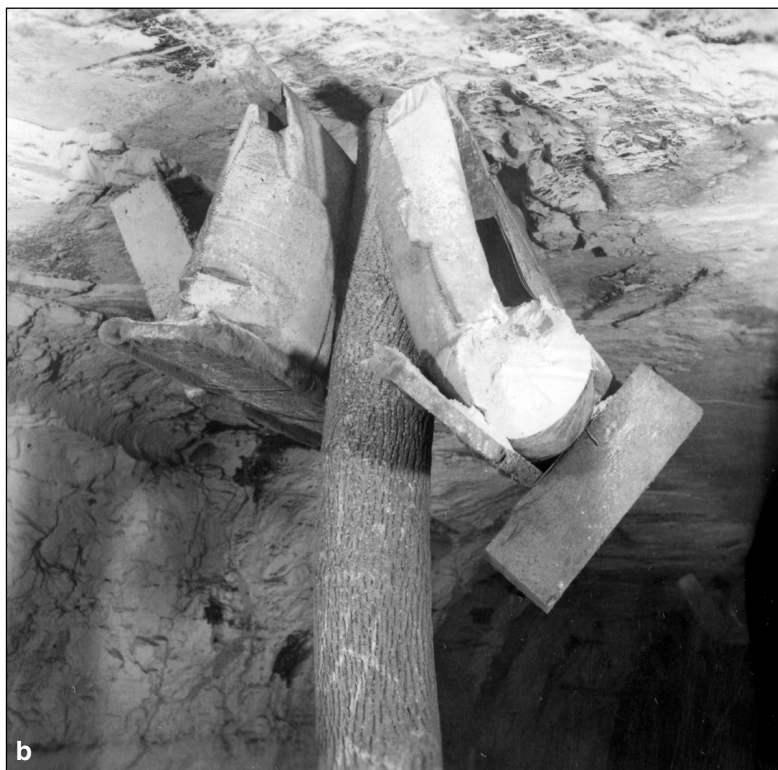
Figure 159 Old Ben Coal Corporation, No. 15 Mine, Franklin County. Quarries began producing 50-pound bags of rock dust, which decreased the labor of installation. Even so, a mine required thousands of bags. The bags were constructed with a small gauge wire that would rip the paper and allow the dust to be dispersed. (a) The center bag has been tripped by hand, but, in an explosion, the air gust would trip the hanging vane, removing the support so that the bag would rip and disperse dust from the barrier above the entry. (b) The platform base would then drop, causing the wire to rip the bag and disperse the dust (Jones 1938).
