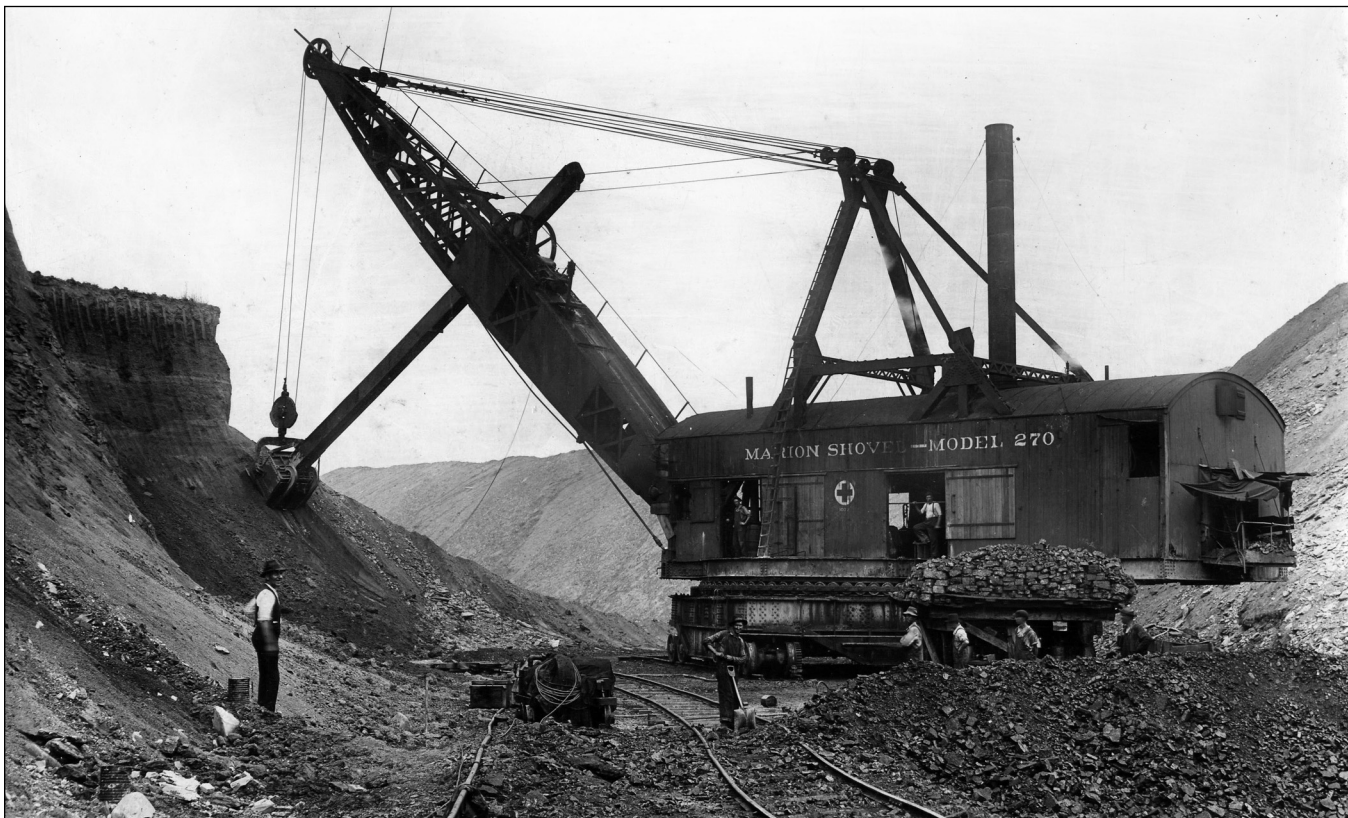
Figure 179 Mine unknown, probably located in Vermilion County. This Marion 270 steam shovel shares many aspects with the Marion 250: a fully revolving shovel with four four-wheeled bogies for mobility. The 5-cubic yard bucket (Historical Construction Equipment Association 2002) was larger and the 90-foot boom longer than the Model 250 (Hollingsworth 1963).
