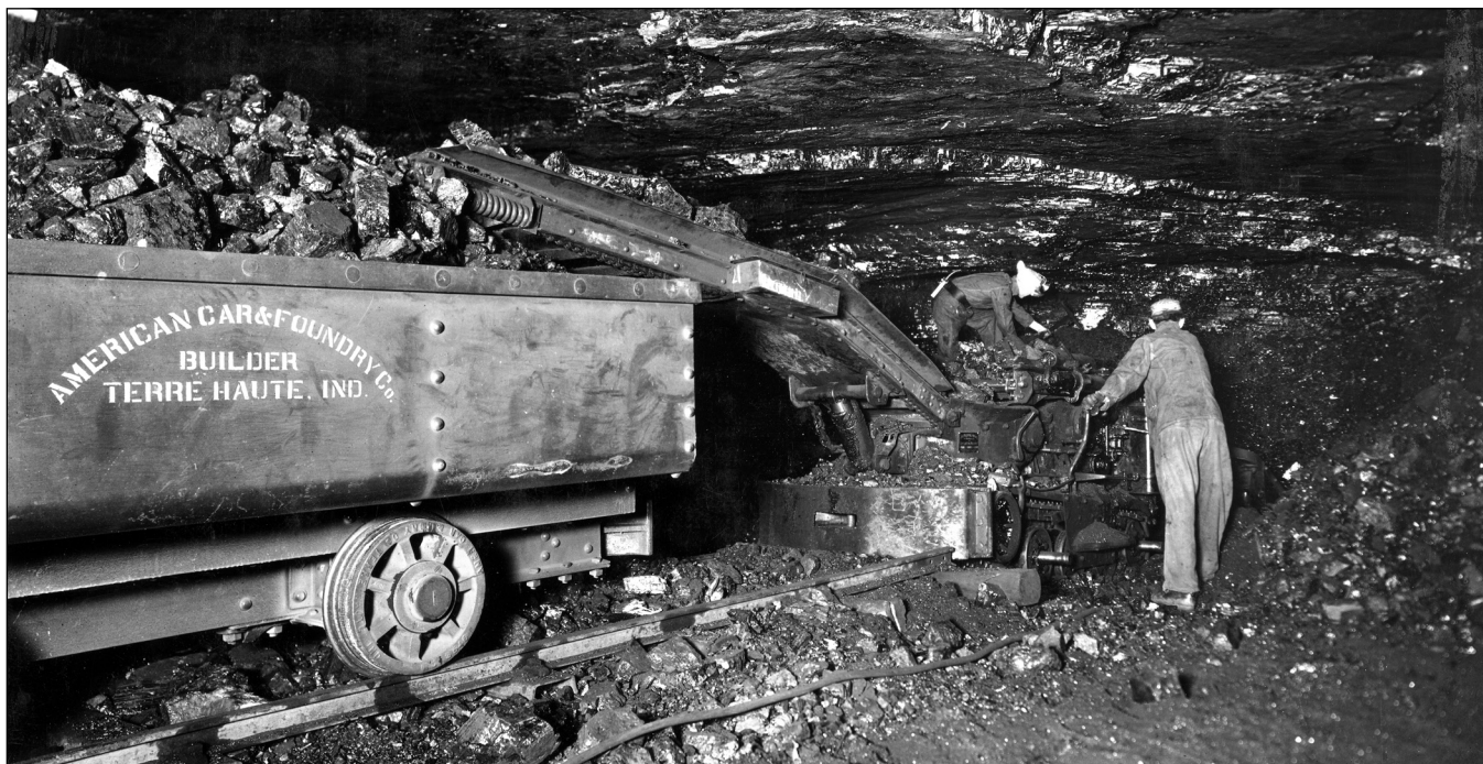
Figure 50 Chicago, Wilmington & Franklin Coal Company, New Orient Mine, Franklin County. The Joy mechanical loader, powered off the trolley using a trailing cable, was versatile, efficient, and reliable. Because it was crawler mounted and not tied to the track, it outperformed hand loading by an incredible margin. These machines became even more efficient when teamed with shuttle cars. Ultimately, they became the loading and conveying portion of continuous mining machines (Ledvina et al. 1992).
