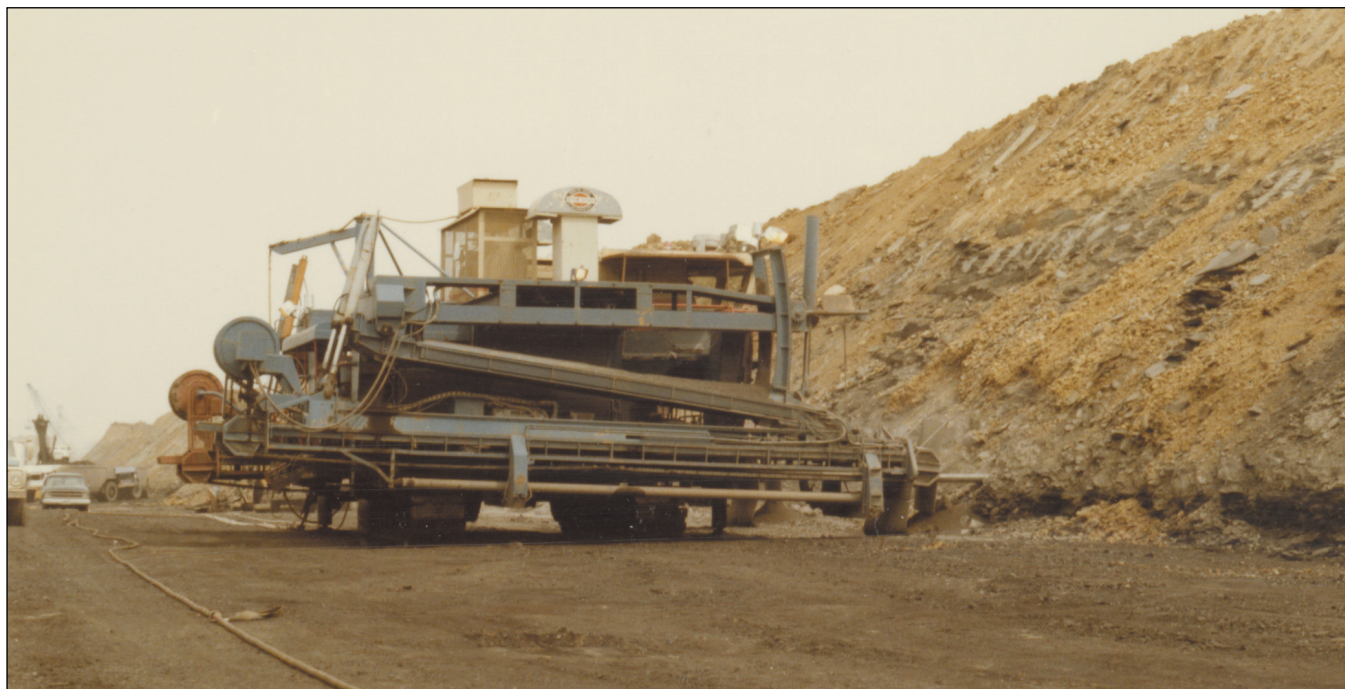
Figure 251 Arch of Illinois, Inc., Captain Mine, near Willisville, Perry County. Horizontal drill holes were often used to shoot the overburden from the coal in Illinois surface mining. At the Captain Mine, these holes were drilled 60 feet into the highwall about 3 feet above the Herrin Coal, ordinarily in the Brereton Limestone.
