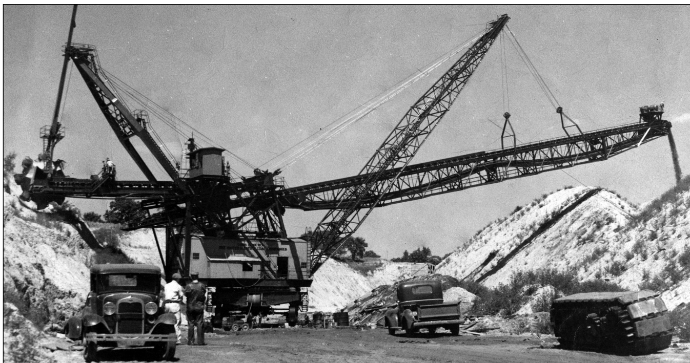
Figure 212 United Electric Coal Company, Cuba Mine, Fulton County. This is the first wheel excavator, pioneered by Frank F. Kolbe of United Electric Coal Company. Kolbe wanted an economical method of moving a great volume of soil and shale and depositing it far enough away to prevent the spoil pile from sliding back into the pit (Hollingsworth 1963). This wheel excavator could deposit to a spoil pile 400 feet away. Bucyrus built the upper portion, which was attached to a Marion dragline base. The machine weighed about 1,000 tons and had an output of 1,000 cubic yards of material per hour. This volume is about five times that of the Marion dragline model that the base was taken from (United Electric Coal Companies 1949).
