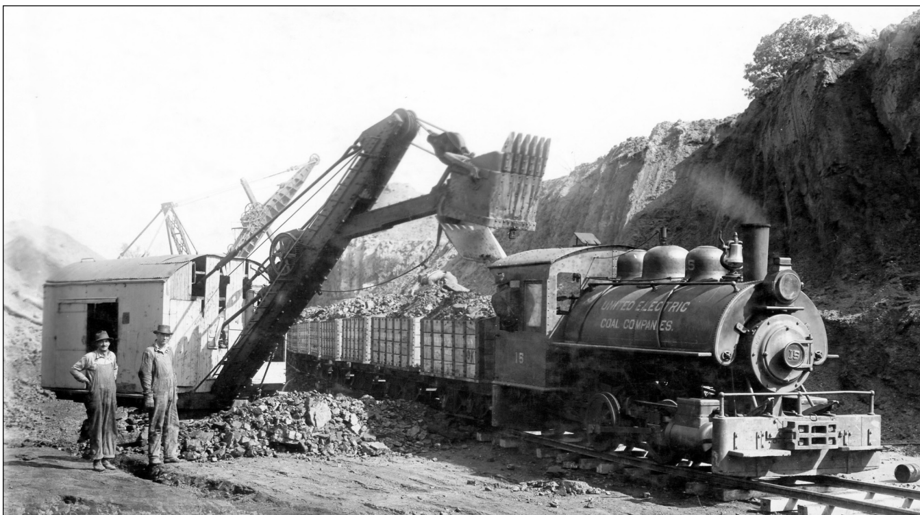
Figure 201 United Electric Coal Company, Vermilion County. A larger shovel in the background (only the boom and dipper stick are visible above the loading shovel) removes overburden while this shovel is used for loading.
