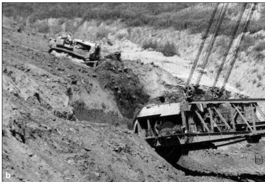
Figure 230 Peabody Coal Company, River King Mine, near Freeburg, St. Clair County. (a) The cutting head of the excavating wheel is shown. The previous cut can be seen above the head, but it is weathered, and the debris has slumped so that the characteristic curved excavation marks are not easily discernible. (b) A bulldozer working in conjunction with the bucket wheel excavator makes an efficient machine even more so.
