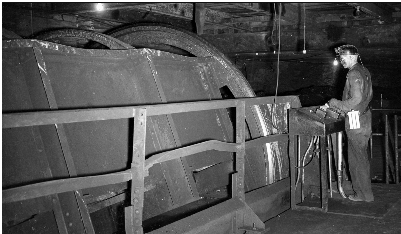
Figure 109 Sahara Coal Company, No. 5 Mine, Saline County. An underground rotary dump weighs and dumps coal cars into an underground hopper. From that point, the coal is fed onto a belt line that carries the coal up a slope entry into the preparation plant (Ledvina et al. 1992).
