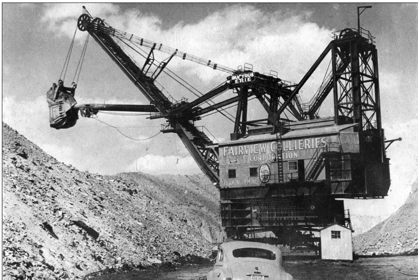
Figure 208 Fairview Collieries Corporation, Flamingo Mine, Fulton County. Bucyrus-Erie 950-B stripping shovel shown at work. This photograph shows the counterbalanced hoist mechanism at the rear of the housing very clearly.
