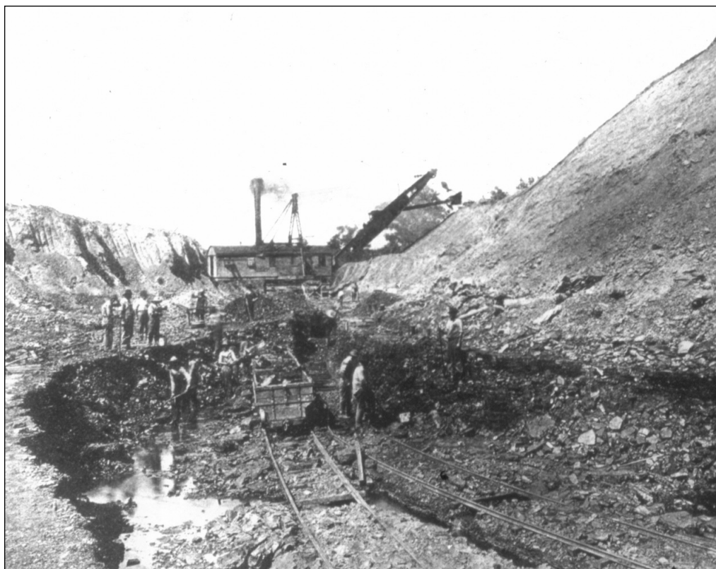
Figure 180 Danville area, Vermilion County. Hand loading was preferable in some mines even when small steam shovels were available. Some coal seams have two or more benches separated by bands of shale, and it was more efficient to leave that shale in the pit. Hand loading of the coals could contribute to the cleaning process by saving time and labor in the sorting sheds.
