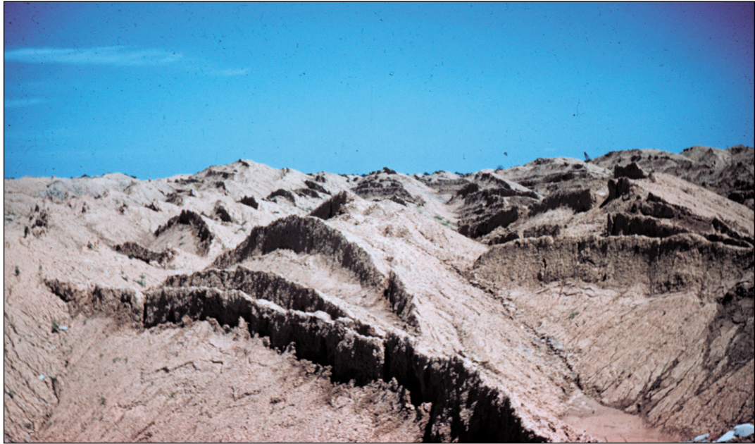
Figure 278 Mine and location unknown. This 1960 spoil pile shows the appearance of unreclaimed surface-mined lands before reclamation laws took effect. Current laws require that overburden be graded within 180 days of coal removal and that no more than four ungraded spoil ridges should exist behind the active pit (Illinois Department of Natural Resources, Office of Mines and Minerals, undated).
