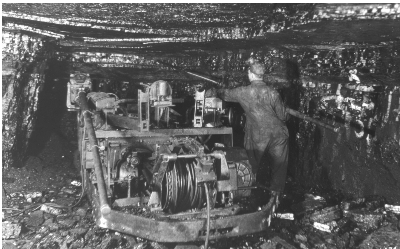
Figure 44 Mine and location unknown. This operator and machine are inserting Cardox or Airdox cartridges.
