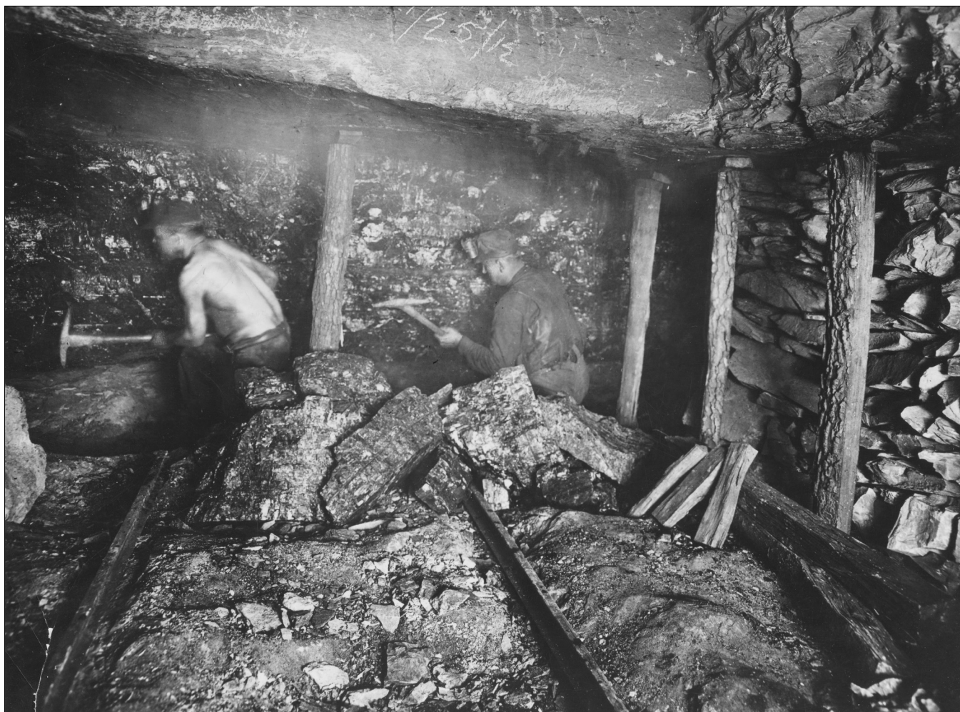
Figure 25 Mine unknown, Grundy or Will County in northeastern Illinois. These miners are undercutting the face of a long-wall mine. The roof is supported by timbers and a rock pack wall (right side).
