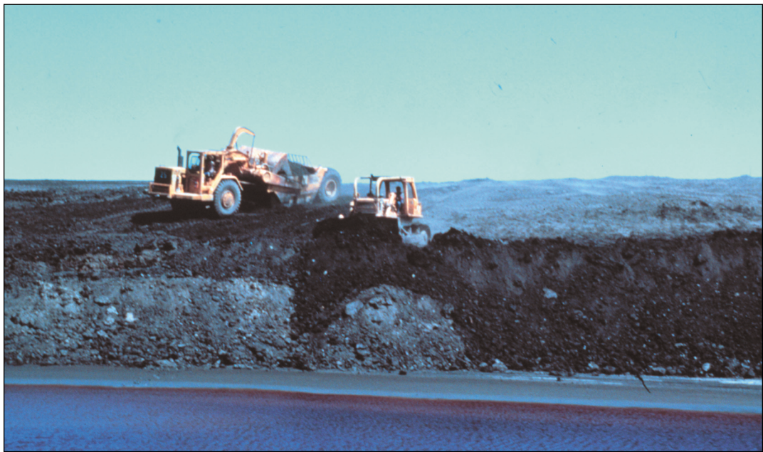
Figure 279 Freeman United Coal Company, Crown No. 1 Mine refuse pile, Montgomery County. Grader and bulldozer smooth out an area under reclamation. Graders and scrapers are necessary tools for removing and stockpiling topsoil and subsoil and for dispersing these soil materials during the reclamation process.
