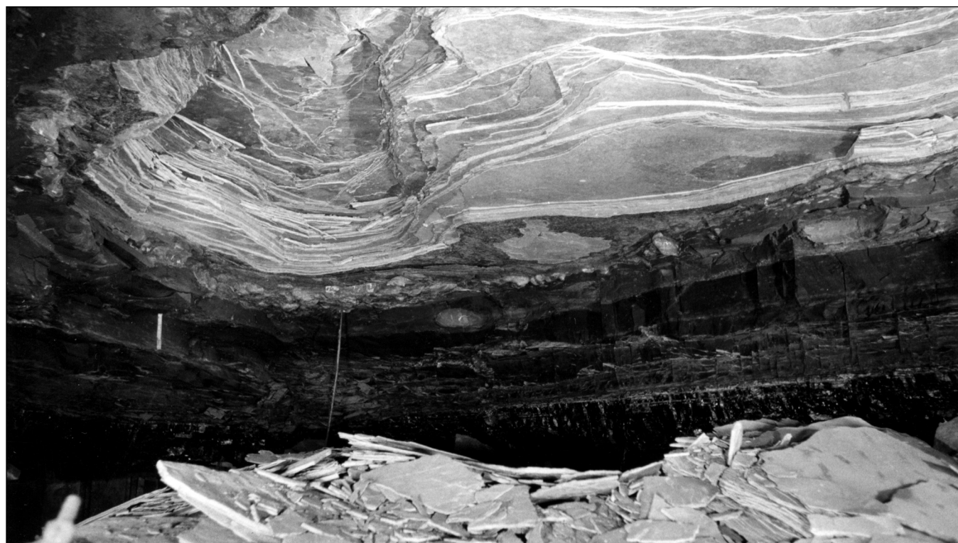
Figure 131 Peabody Coal Company, No. 10 Mine, Christian County. This roof fall shows about 3 feet of thin beds of sandstone interbedded with thin bands of shale, which kept the sandstone layers from adhering to each other. Below the sandstone is a layer of limestone that varied from 6 to 18 inches. About 3 feet of black shale was between the coal and limestone.
