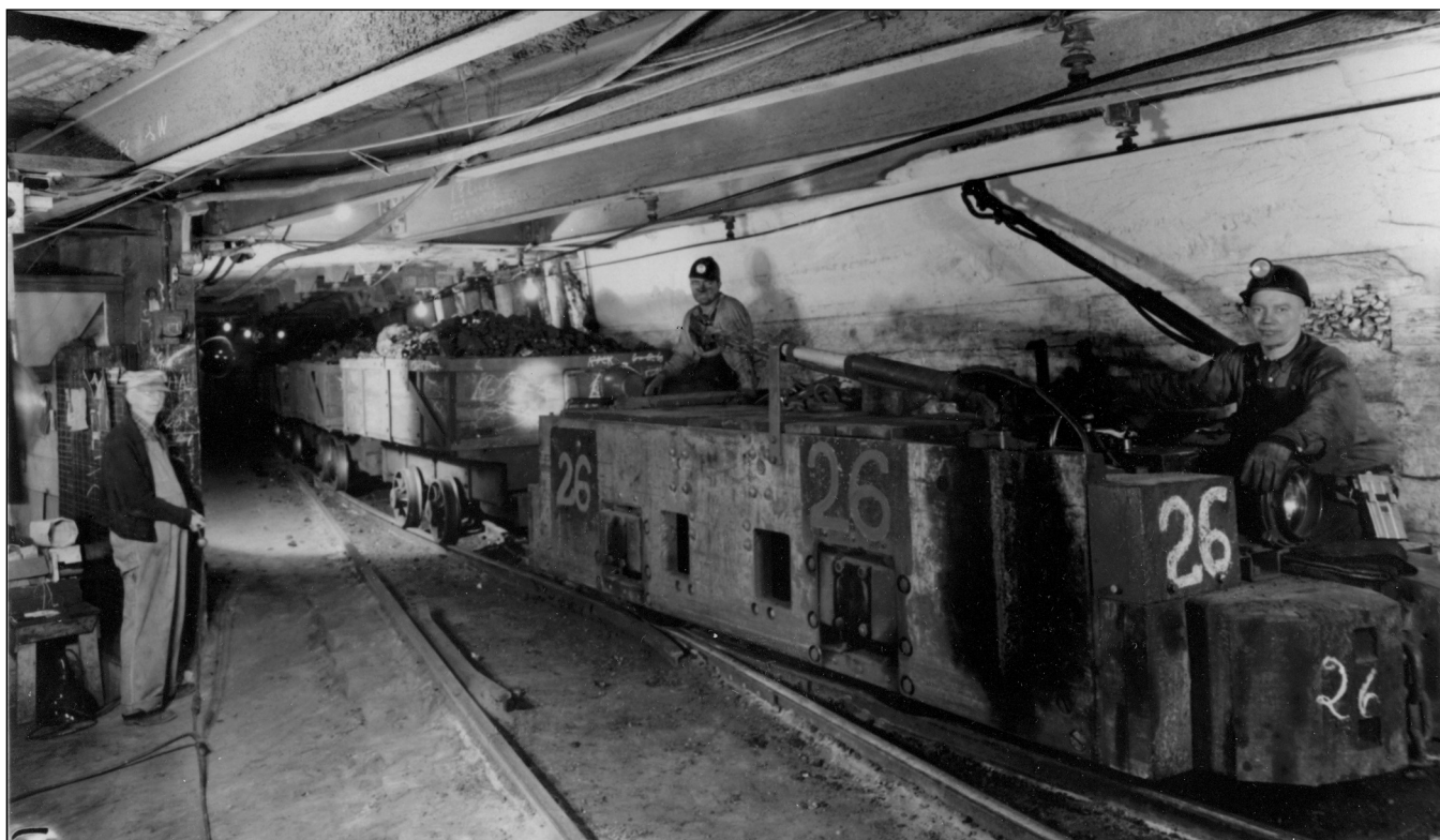
Figure 71 Bell & Zoller Coal Company, No. 2 Mine, near Zeigler, Franklin County. Main line motor hauling a loaded trip of mine cars to the shaft bottom. The motorman is in front and is assisted by a trip rider. The dispatcher is at left (Ledvina et al. 1992).
