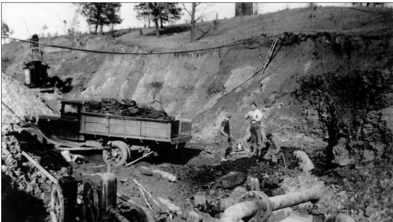
Figure 200 Kedas Mine near Danville, Vermilion County. Even with the appearance of such large machines, smaller mines continued to operate as they had in the 1920s. The truck is a 1934 Ford. This photograph shows safety hazards that would never be allowed in a pit today, including the ladder on the highwall to exit the pit and the draped cable across the pit that is either an electric cable or a water sump hose.
