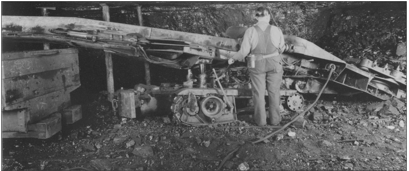
Figure 57 Bell & Zoller Coal Company, No. 2 Mine, near Zeigler, Franklin County. A Joy 11BU loading machine in action. Loading machines grew in size and complexity with increased reliability and greater capacity (Ledvina et al. 1992).
