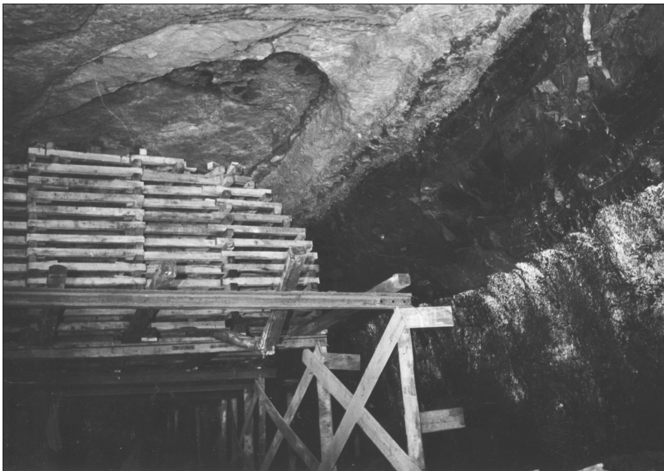
Figure 147 Peabody Coal Company, No. 10 Mine, Christian County. Cribbing was used here to stabilize an area sensitive to roof falls, a major haulage route. Steel and wood are used to construct a frame for shuttle cars to drive under and to support the cribbing that in turn supports the roof (Coal Section mine notes).
