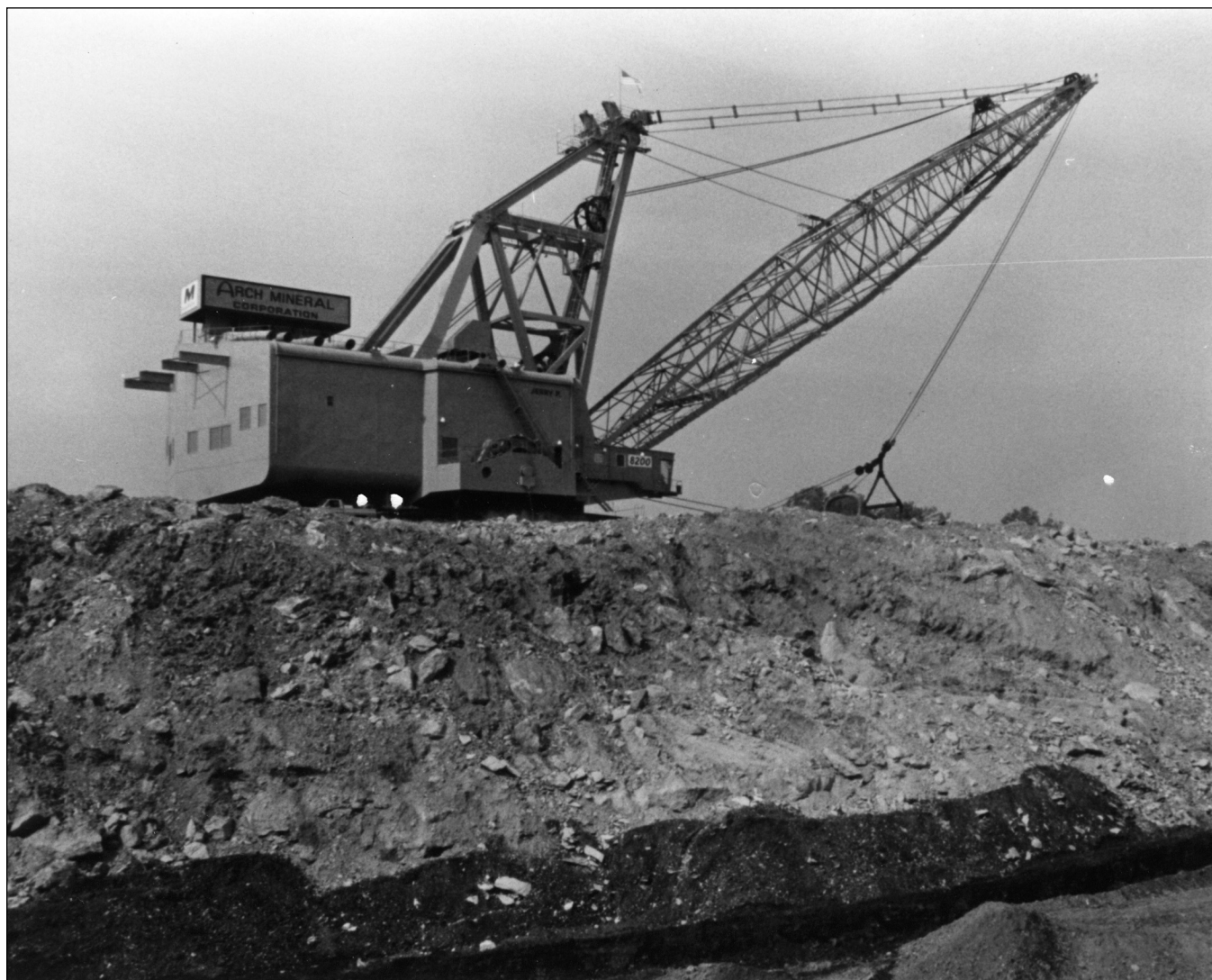
Figure 244 Southwestern Illinois Coal Corporation, Streamline Mine, near Percy, Randolph County. Here is an 18-story tall walking dragline, a Marion 8200. This dragline weighed 4,450 tons and could manage a 65- to 95-cubic yard bucket (Historical Construction Equipment Association 2002), depending on the type of material to be excavated. The dragline used electrical power (7,000 horsepower) equivalent to the needs of a city of 15,000 people (Ledvina et al. 1992).
