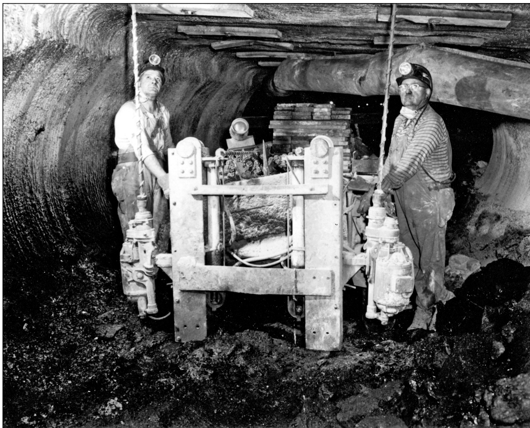
Figure 140 Bell & Zoller Coal Company, No. 3 Mine, near Zeigler, Franklin County. This photograph shows an early dual-boom roof bolting machine. The operators of this machine work close to unsupported roof. The curved side walls indicate that a boring-type continuous miner excavated this room, and speed was essential to keep up with the advance rate of the mining machine.
