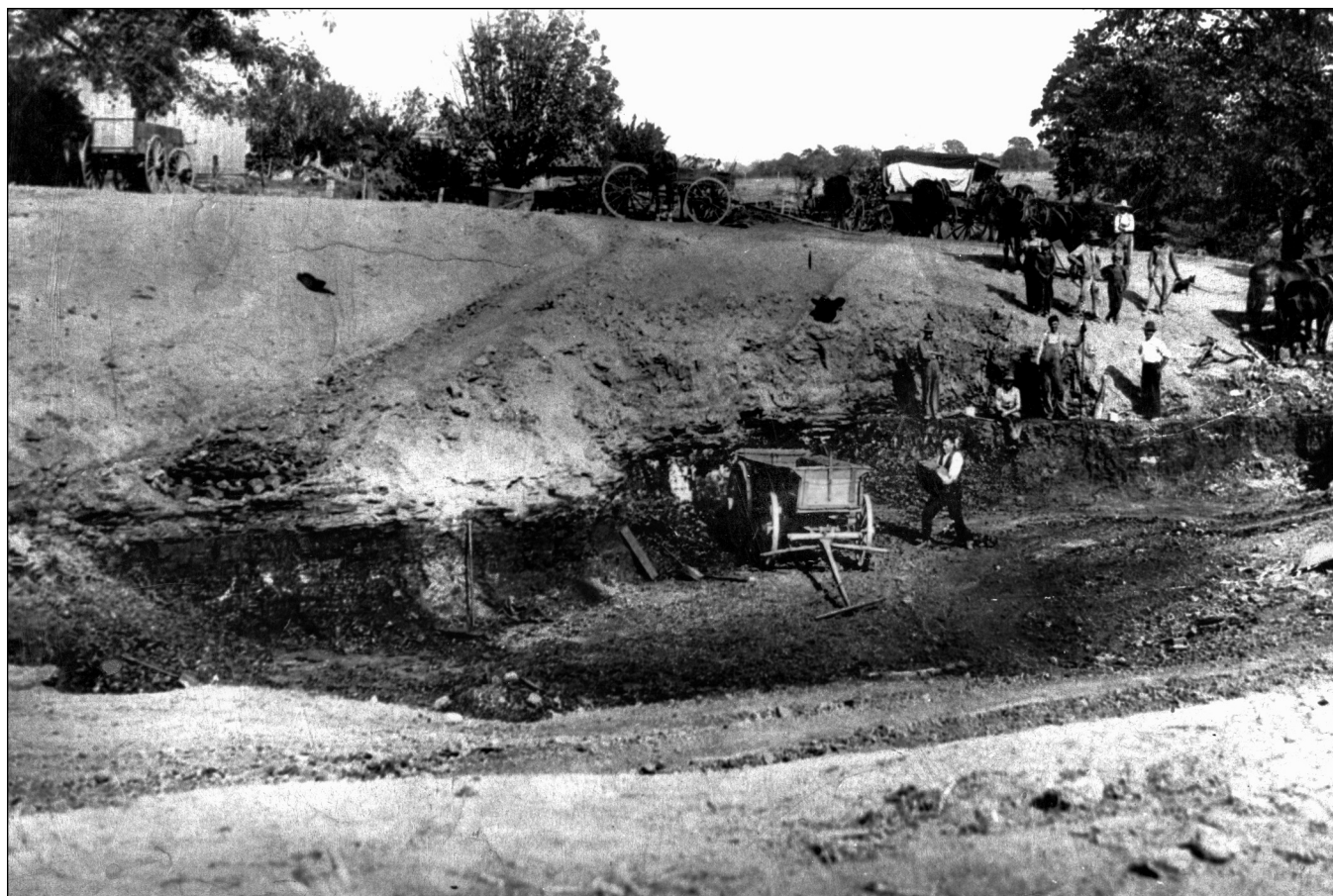
Figure 168 A typical early mine. Coal is dug out along the outcrop with picks and shovels, loaded into wagons, and hauled to market or used for heating in homes close to the mine. Surface mining by this method was practiced for more than 100 years, from the earliest mining in the 1830s.
