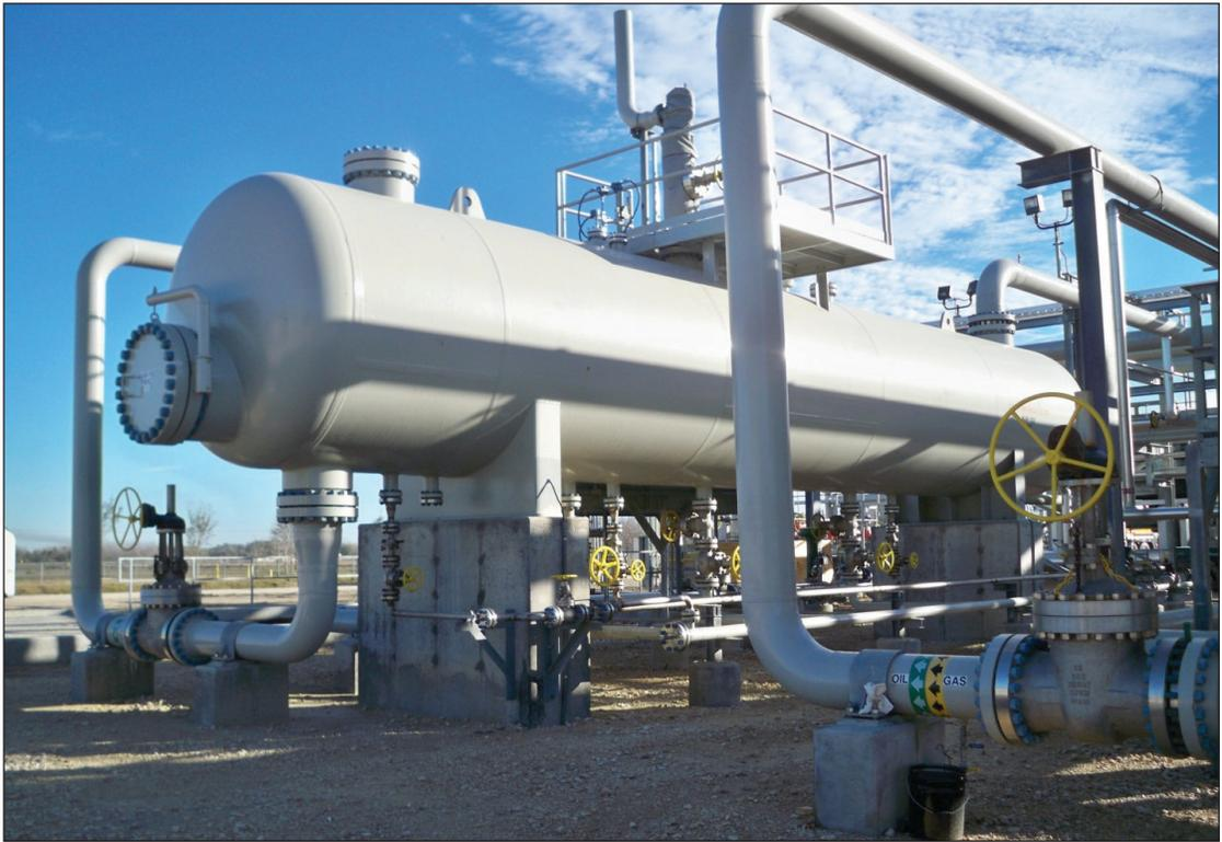
**Figure 1** Typical horizontal free water knockout vessel. The horizontal slug catcher and demulsifier vessels are similar in appearance. Photograph courtesy of Denbury Onshore.
