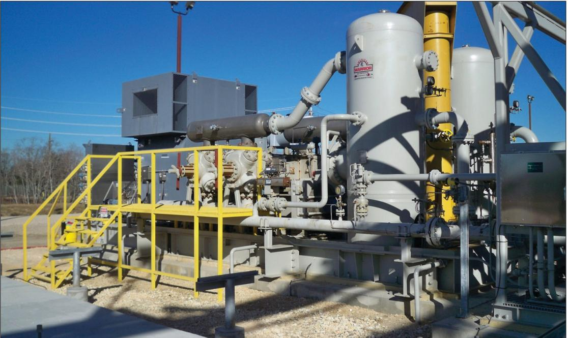
**Figure 2** Typical vertical vessel high-pressure suction scrubber and compressor. Typical low-pressure suction scrubbers are similar in appearance. Photograph courtesy of Denbury Onshore.
