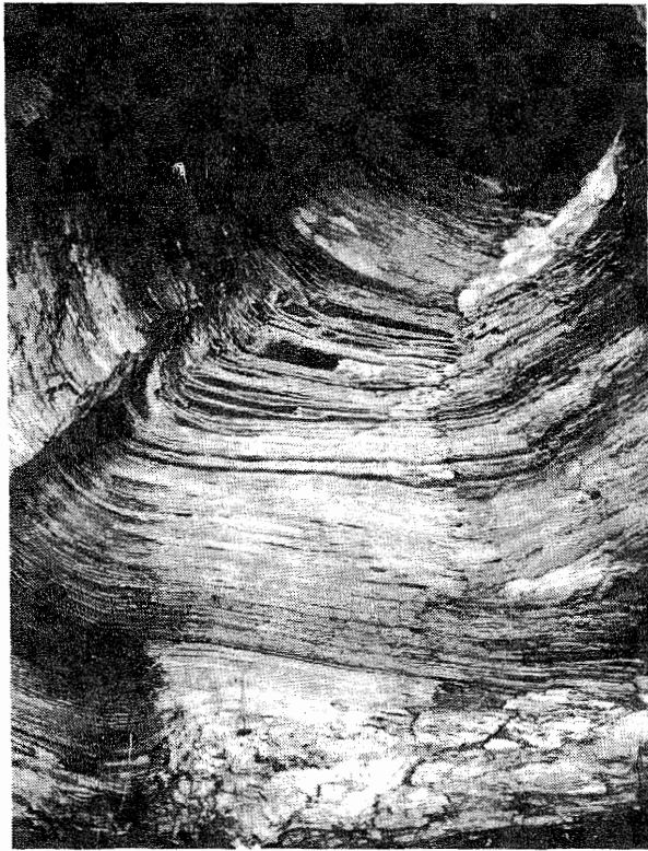
Figure 20. Roof fall in planar-bedded sandstone of the Energy Shale Member. Bedding surfaces are coated with mica and coalified plant fragments. No prominent joints are visible. Sandstone failed and broke almost straight up along the pillar rib. Location: "Quality Circle," near Walshville channel, mine C.
