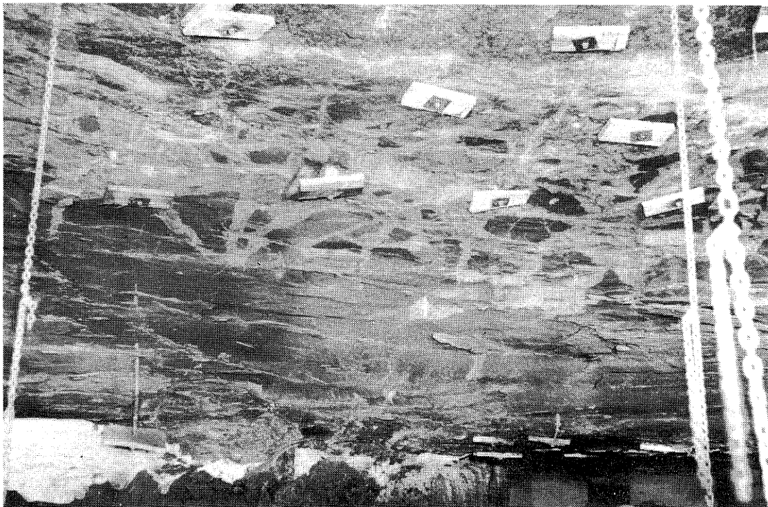
Figure 87. Syneresis cracks and mottled shale a few feet above Herrin (No. 6) Coal. Mottled shales are very weak strata in which standard roof bolts cannot be anchored easily. Original bolts had been set into the mottled shale, but were pulled out as the roof failed. Location: mine E in southwestern Illinois.
