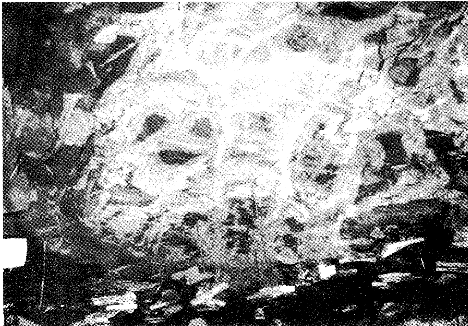
Figure 80. Mottled shale with syneresis cracks in greenish medium-gray shale, above very dark gray shale, probably Lawson Shale (with syneresis cracks) above Anna Shale. Note roof bolts hang out bare; the soft shales have fallen because of moisture slaking; in the center of roof fall, bolt anchors even have fallen out. Location: mine F in east-central Illinois.
