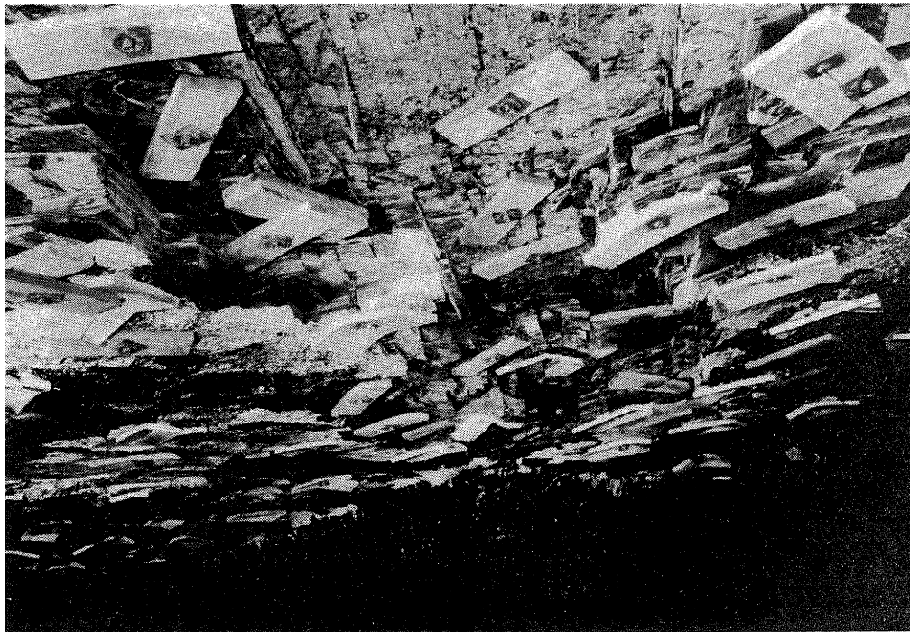
Figure 70. Prominent set of joints in black fissile shale (Anna Shale). Slabs, separated along bedding planes and joints, fall out between the roof bolts. Location: mine N, west-central Illinois.
