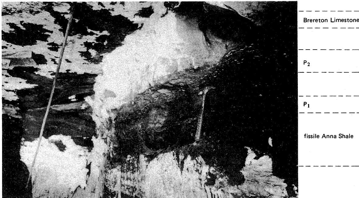
Figure 66. Black shale-limestone roof in mine A (west-central Illinois). The Brereton Limestone (appears white because of rock dust) is two feet (0.6 m) thick and overlies thick strata of Anna Shale. The two layers of phosphatic nodules ( P_1 and P_2 ) in the upper, poorly bedded, weak, very dark shale are clearly shown; the black fissile ("slaty") lower shale above the coal is covered by rock dust (white). Total thickness: three feet (0.9 m).
