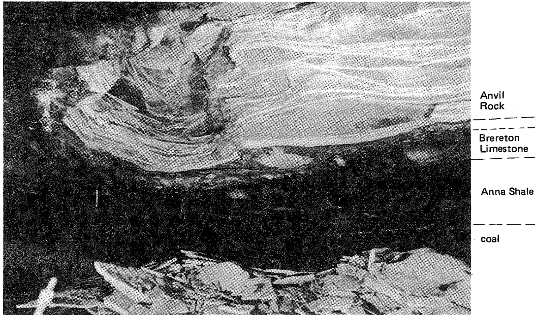
Figure 21. Roof fall in a sequence of Anvil Rock Sandstone (planar-bedded, light gray siltstone and sandstone), Brereton Limestone (gray, cloddy limestone with nodules and concretions), Anna Shale (weak, slightly mottled upper portion and well-bedded, well-jointed, fissile lower portion), and Herrin (No. 6) Coal. Roof fall extends up to a tabular, plant-debris-coated bedding surface of sandstone. Planar-bedded sandstones and siltstones of the Energy Shale often fail in the same manner. Location: Western Shelf, west-central Illinois, mine N.
