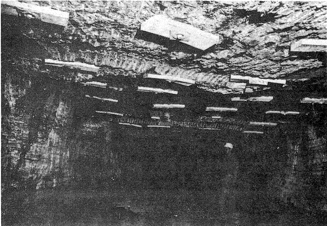
Figure 17. Top coal left in an entry cut by a ripper type of continuous miner. Although the cutting height is variable and more coal can be produced, the hazard of rib rashing along straight vertical ribs is greater (left side of photo).
