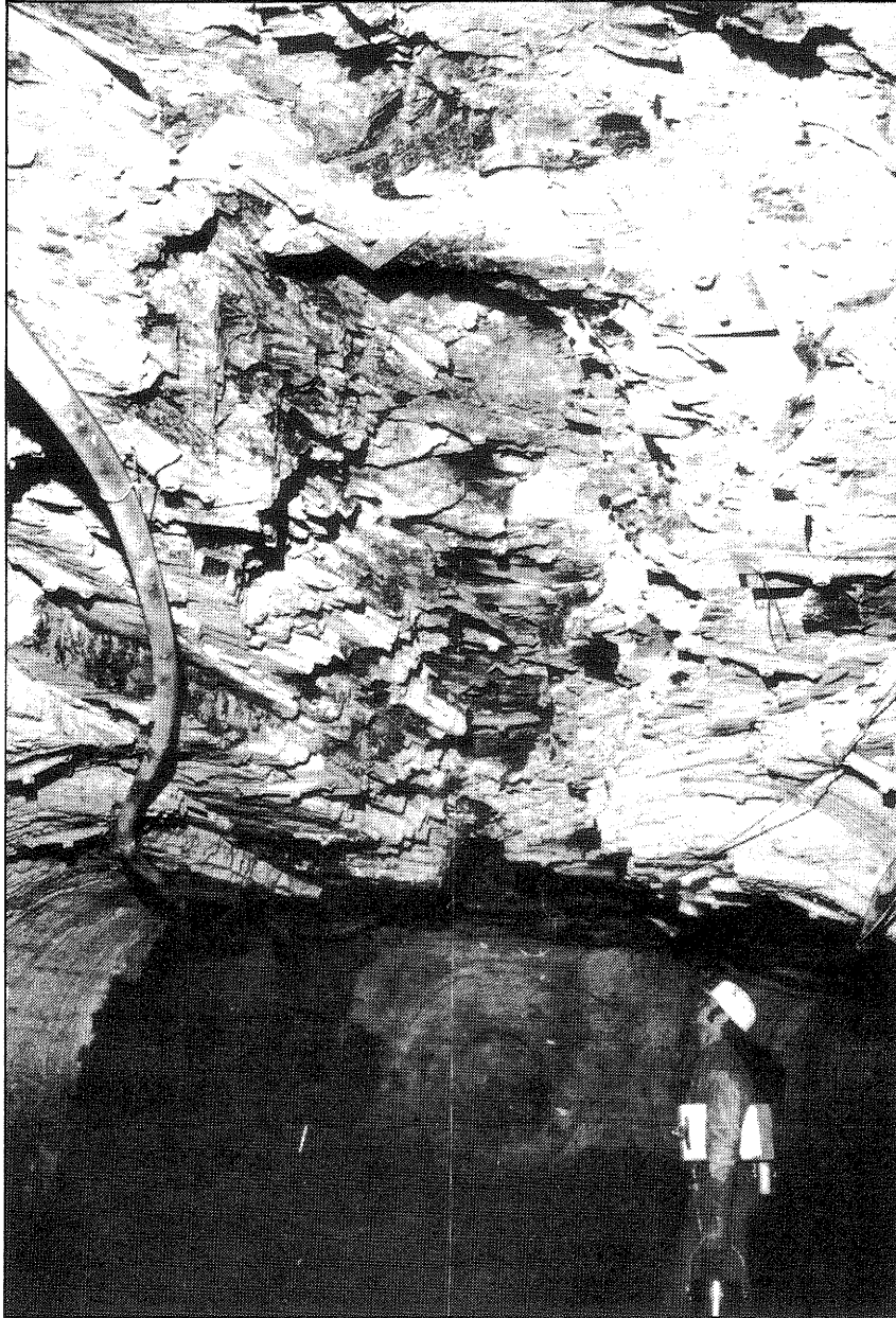
FIGURE 43. North-south "kink zone" caused by large horizontal compressive forces , in roof of Old Ben Mine No. 24, Franklin County, Illinois (Bauer and DeMaris, 1982).
