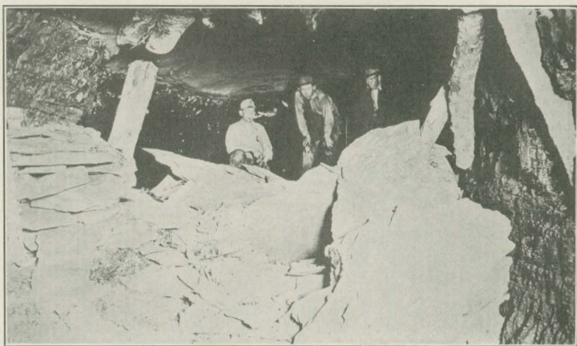
FIG. 13. Roof-fall in entry
