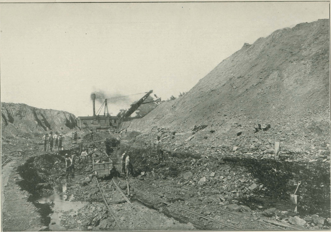
FIG. 29 Stripping-mine coal face
