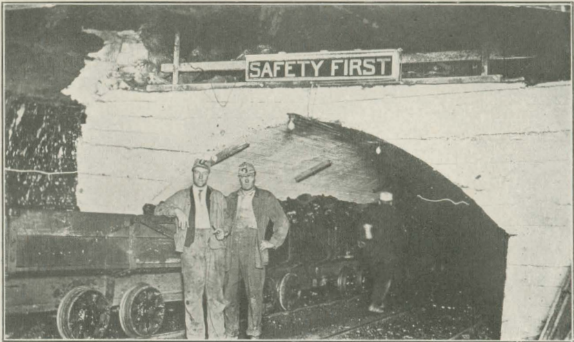
FIG. 17. Inby end of concrete-lined bottom
