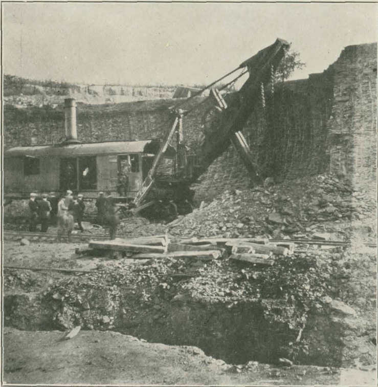
FIG. 24. Steam-shovel digging shale overburden
