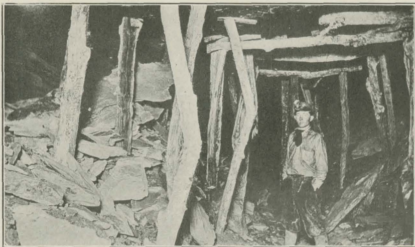
FIG. 11. Destruction of timber by crushing
