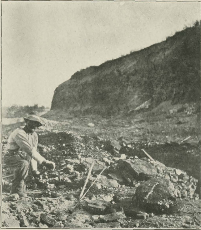
FIG. 25. Drilling hole for blasting at stripping-mine
