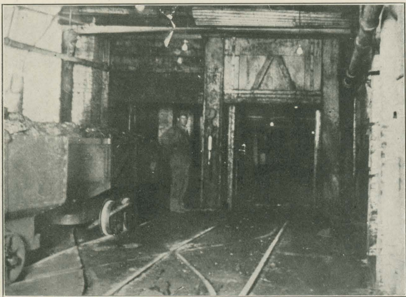
FIG. 19. Typical caging-place at shaft-bottom
