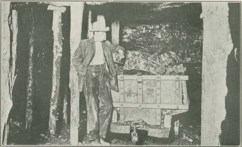
FIG. 14. Method of propping near face of room
