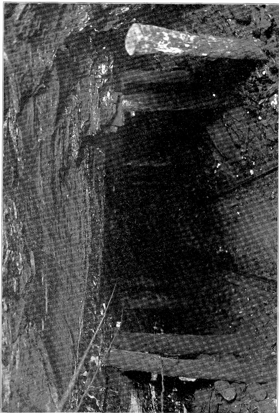
FIG. 18.—Photo showing nature of bedding in black shale roof. (Courtesy Madison Coal Corporation.)
