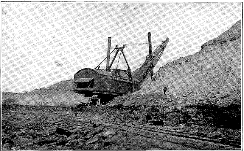
FIG. 26.—Fischer Fuel Co., stripping mine, Millstadt, showing method of removing overburden. (Photo by Fischer Fuel Co.)
