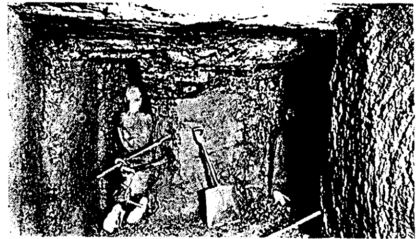
FIG. 15. Shearing the ribs in District VII.
