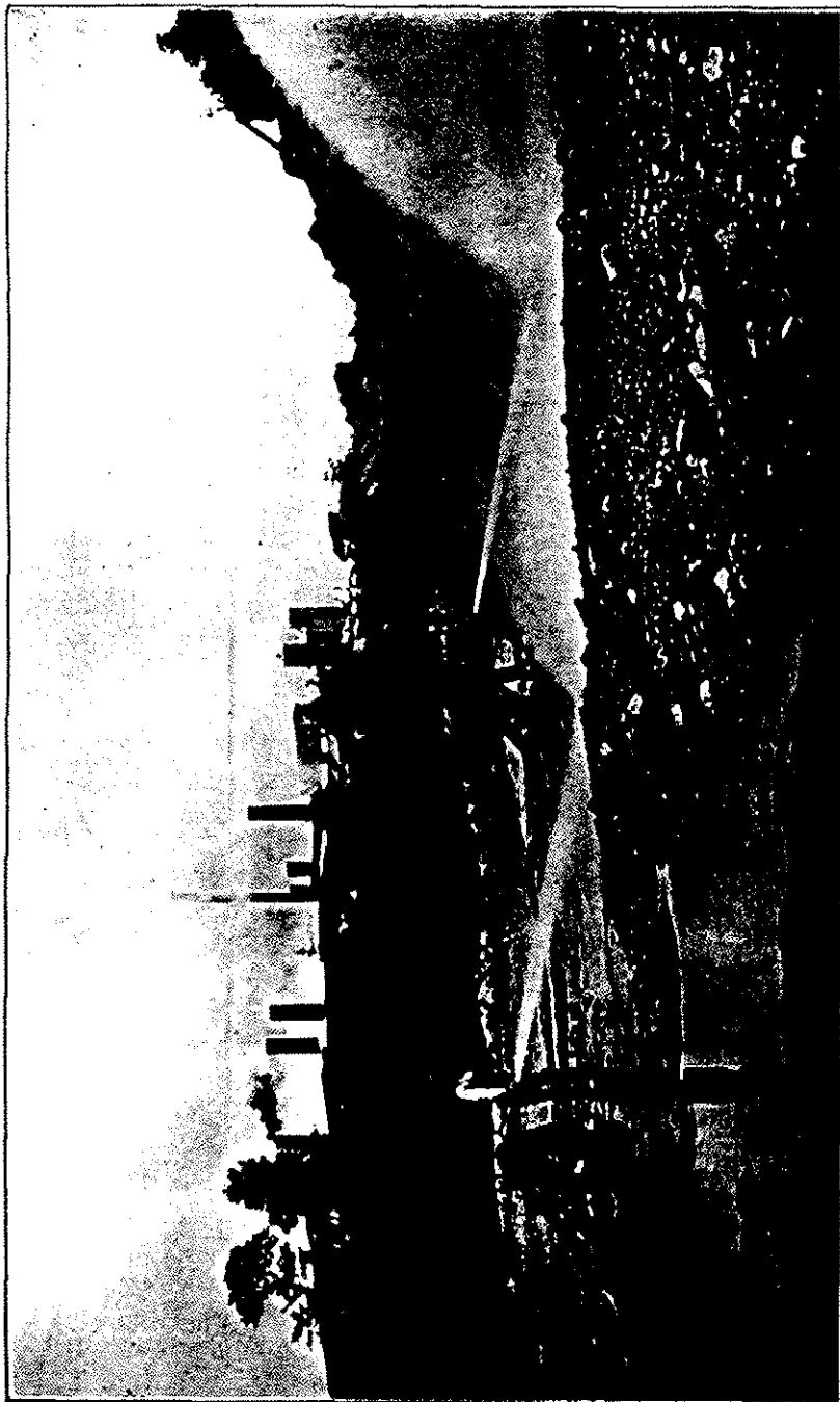
FIG. 28. Removing top soil with hydraulic monitors
