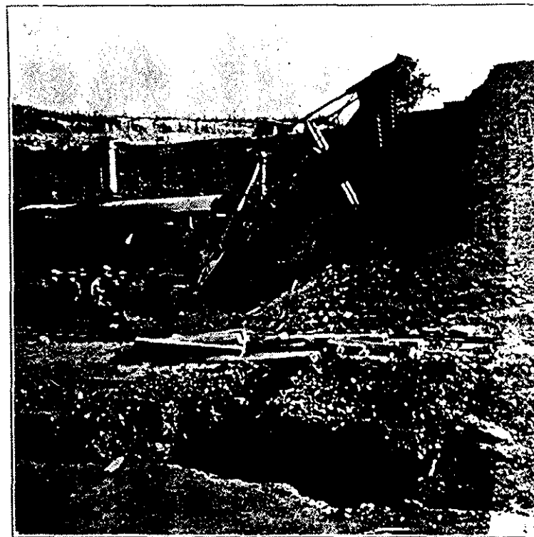
FIG. 29. Steam-shovel digging shale overburden
