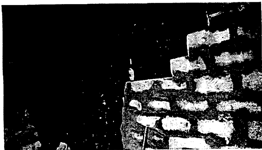
FIG. 50. Latch in rib dug to receive stopping
