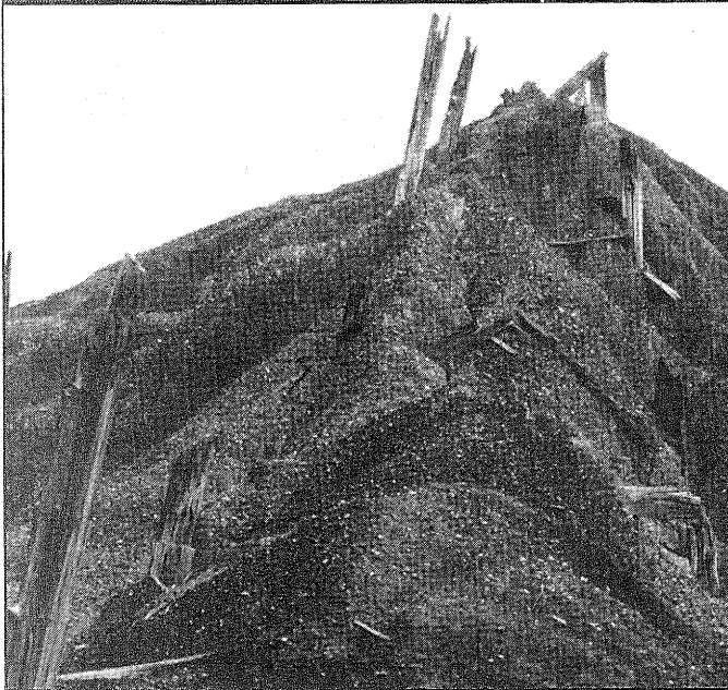
Figure 4 Top: Tipple and mine gob pile at Dalzell. Middle: Remains of a wooden trestle protrude from a pile of preparation gob at Dalzell. Bottom: Two piles at Standard showing typical skewed-cone shape of gob piles.
