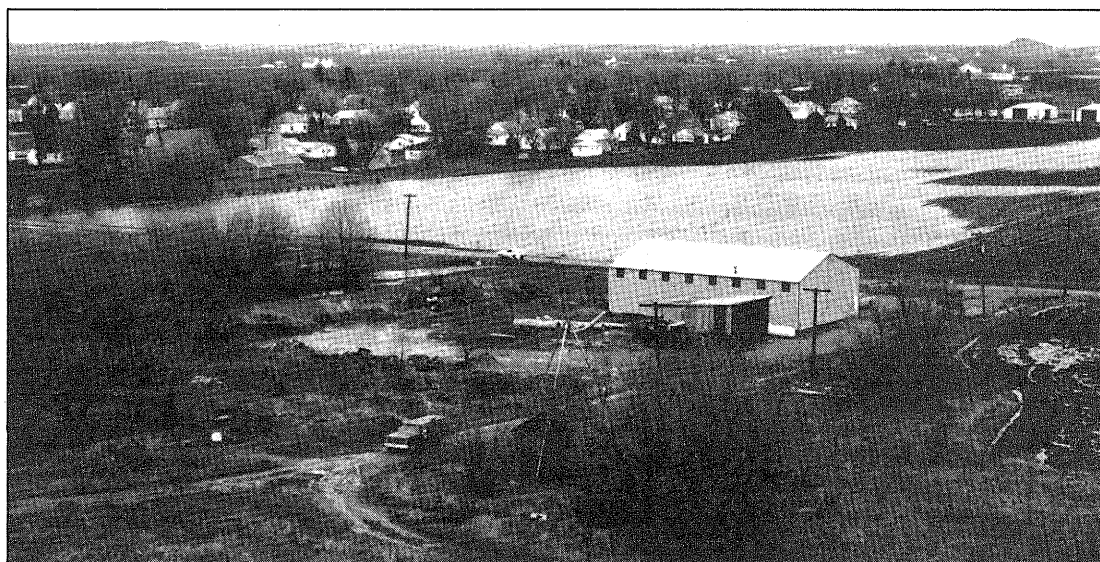
Figure 16 Mud from piles of mine gob at Standard filled a drainage ditch, causing repeated flooding of a nearby field; septic tanks adjacent to this ponded field overflowed (photo taken in spring of 1982).
