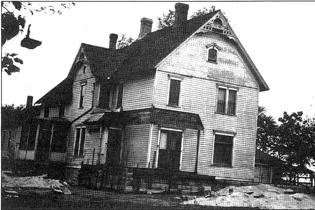
Figure 19 At this house near Coal City, a sag developed over a longwall mine 125 feet underground (Young, 1916). The entire house dropped, but the porch dropped 9 inches more than the rest of the house. Sags in the historic Longwall District stopped developing long ago.
