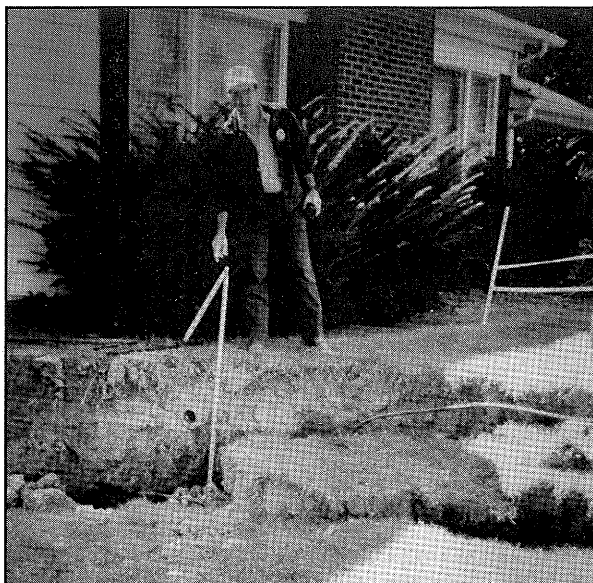
Figure 7 Photograph and cross section of a typical pit subsidence event (after Wildanger et al. 1980).
