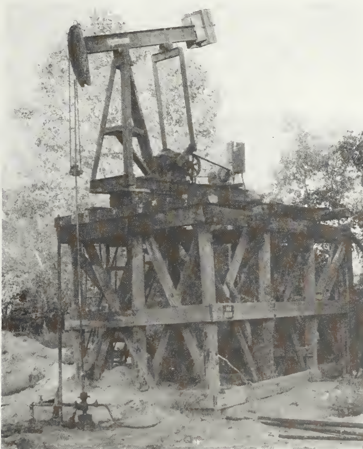
Figure 32 The Mary Heil no. 9 oil well, at Schuh Bend, Stop 7 (photo by W.T. Frankie).
