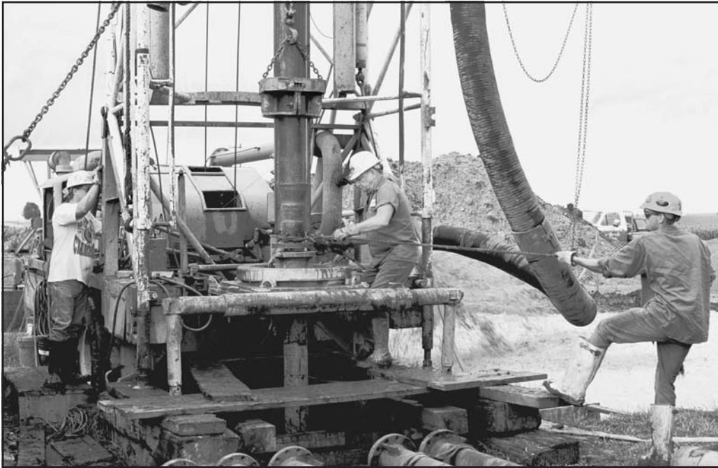
Figure 42 Workers drill a small-diameter water well in Champaign, Illinois.
