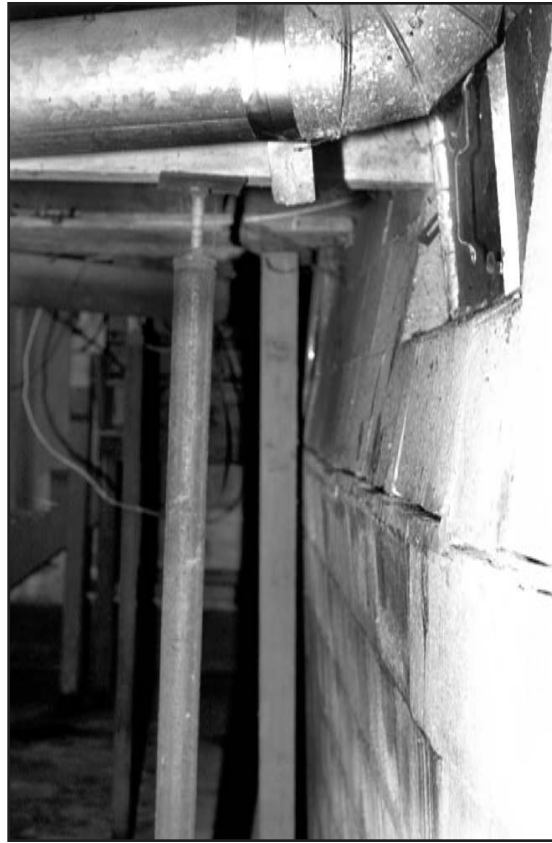
Figure 27 The wall of this building in Christian County was damaged by swelling soils. Note the inward bowing of the wall. (Photo by Bob Bauer.)
