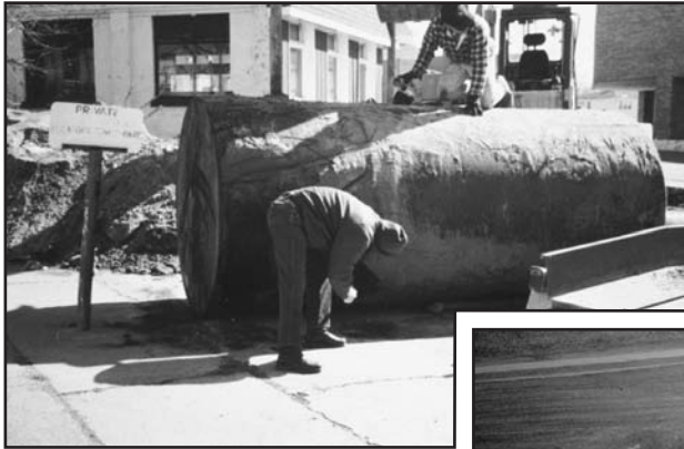
Figure 2 An exhumed tank is examined for leaks. Underground storage tanks usually contain gasoline or chemicals. (Photo by Anne Erdmann.)
