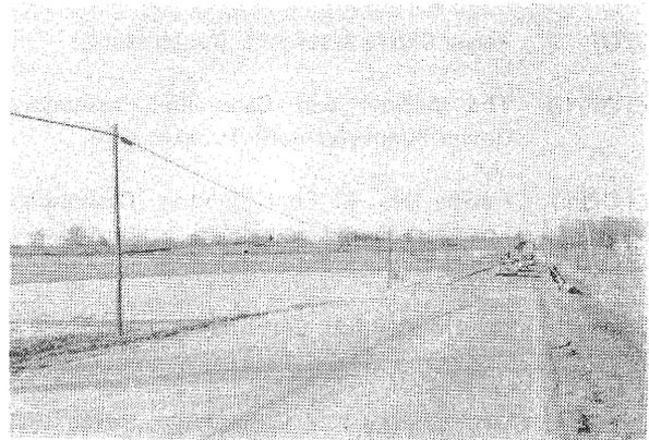
Figure IL-32. Subsidence damage to Illinois Route 13 and adjacent fields, west of Harrisburg, Illinois, above abandoned Mine No. 16, Sahara Coal Company. View to east. Road is being regraded, and ridges either side of cars are gravel.
