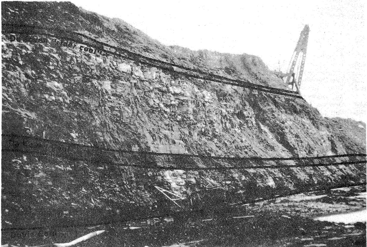
Figure IL-31. Highwall, Will Scarlet Mine. Davis Coal is exposed at the base of the pit, De Koven Coal is about 15 feet (4.5 m) above base of highwall, and 1-foot (0.3 m) coal rider is near the top of the highwall. Note: variation in thickness of interval between the De Koven and "De Koven rider" Coals apparently is due in part to the relatively greater compactibility of shale where the dominant lithology changes from sandstone to shale elsewhere in highwall.
