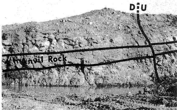
Figure IL-20. Channel phase, Anvil Rock Sandstone, high wall of Eagle Surface Mine. The Brereton Limestone has been locally removed by stream erosion and is replaced by channel-fill deposits of the Anvil Rock Sandstone. At other localities, channel-fill deposits locally replace the underlying Herrin (No. 6) Coal. A small fault (about 1 foot [0.3 m] displacement), which may be related to the nearby Grindstaff Fault (fig. 1L-19), extends diagonally across the highwall.
