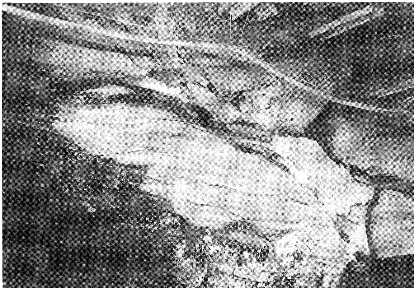
Figure 6. An example of large sandstone-filled rolls common in area of example C. The coal is complexly split and interfingers with the finely laminated sandstone filling the roll. Sandstone shows much internal deformation caused by slumping or differential compaction. Note that miner has been forced to take a large amount of rock with the coal, resulting in irregular roof. Width of view is about 12 feet (4 m).
