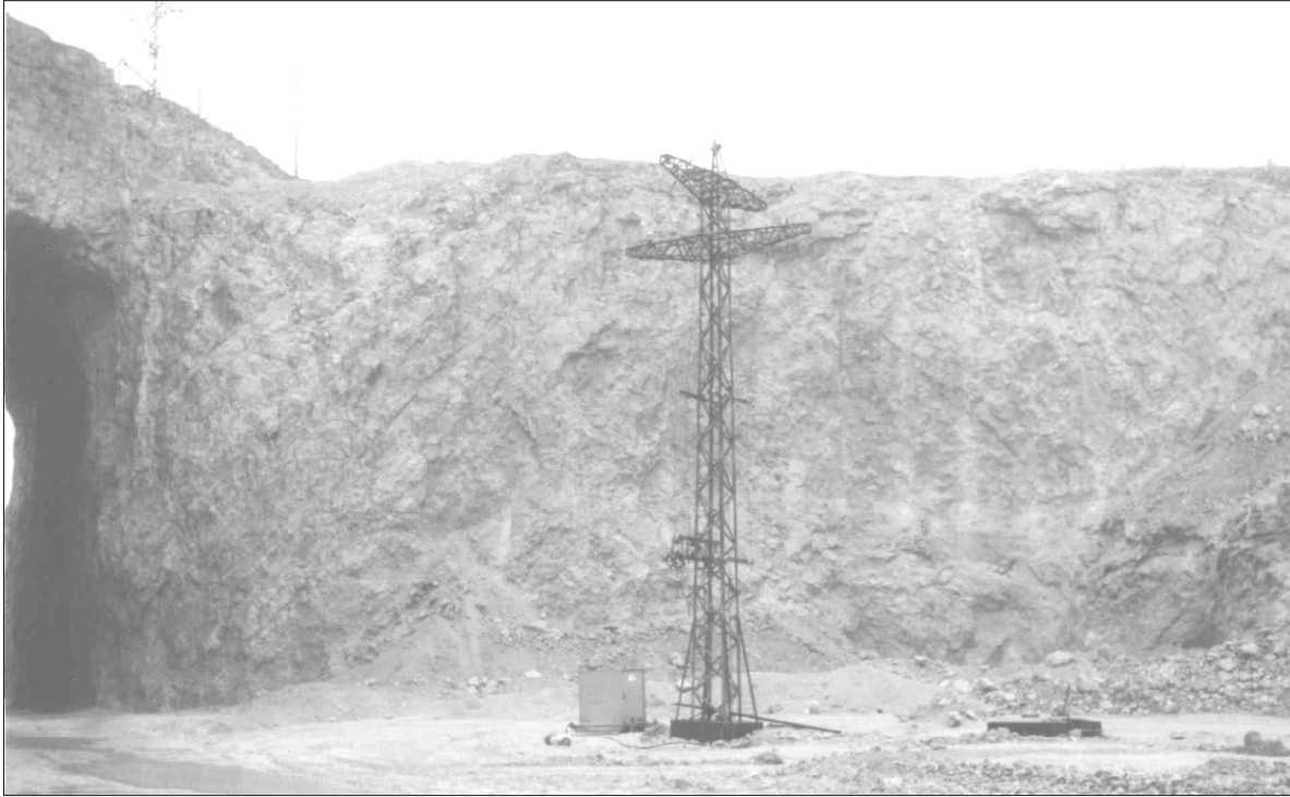
Figure 23 Dip reversal at south edge of upper reef core located below old ramp just west of the main tunnel, main level, Northwest Pit, Thornton quarry (Photo taken in 1974). Weakly defined strata may be seen dipping in opposite directions on either side of the power-line tower near center of photo.
