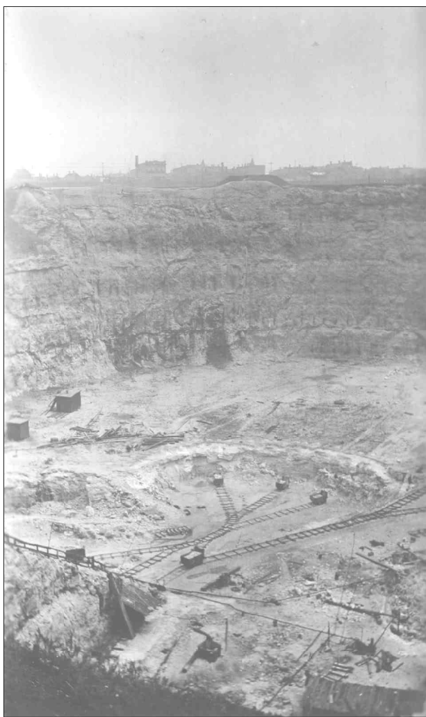
Figure 6 East wall of Stearns Lime and Stone Company quarry. Rock was loaded by hand into quarry cars, which were then pushed along tracks to the base of the incline in the lower left corner of photo. Cars were then pulled by cable up the incline to the kilns. (Photo taken in 1907 by E. F. Burchard, No. 436; Courtesy of the U. S. Geological Survey)
