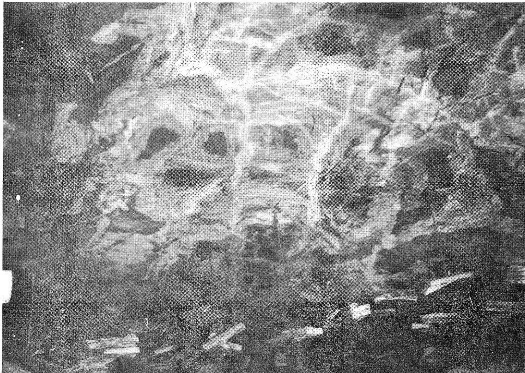
Figure 29. Mottled shale with syneresis cracks in greenish medium-gray shale, above very dark gray shale, probably Lawson Shale (with syneresis cracks) above Anna Shale. Note roof bolts hang out bare; the soft shales have fallen because of moisture slaking; in the center of roof fall, even bolt anchors have fallen out. Location: a mine in east-central Illinois.
