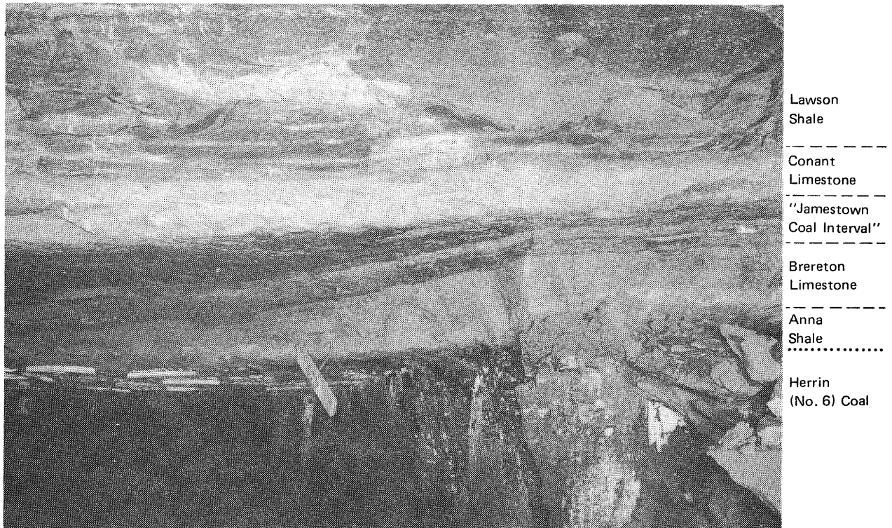
Figure 27. Wedging relationship of roof rock layers; both the Anna Shale and the Brereton Limestone pinch out (toward left side of photo). The "Jamestown Coal interval" has thin coal streaks and contributes to bedding separation. The overlying Conant Limestone is too thin to bridge stresses from one pillar to the next. The Lawson Shale is soft and mottled and contains numerous low-angle shear planes and syneresis cracks. Location: mine A, west-central Illinois.
