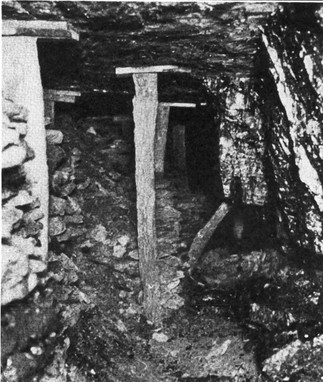
Figure 10. Longwall face with packed rock to left, props and solid coal face to right. This is the working area for the miners, showing same setting as figure 9. Andros 1915 Figure 27.
