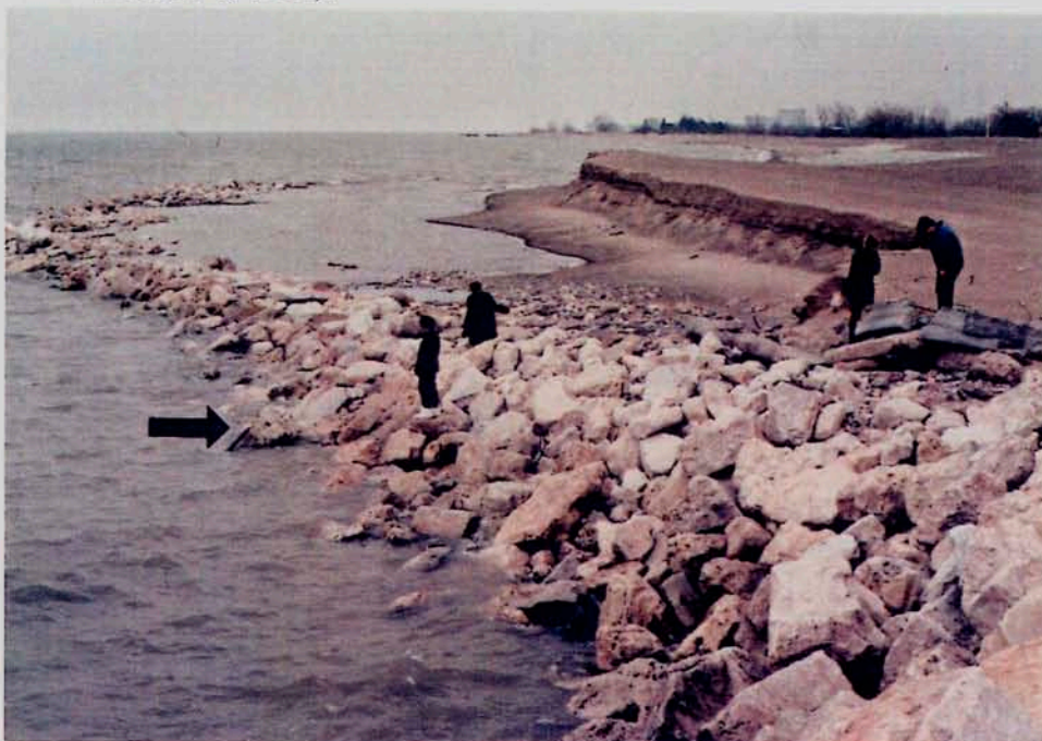
Figure 2-17 Same view of the riprap six months later in April 1990 showing the degree of riprap subsidence and landward erosion (Photo date April 13, 1990).
