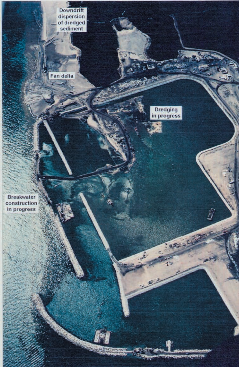
Figure 1-4 Oblique aerial view of the North Point Marina construction site on September 14, 1988 looking toward the south. Sediment dredged from the marina basin is being discharged by slurry pipe to create the fan delta. The fan delta reached its maximum lakeward extent within three months after this photograph.
