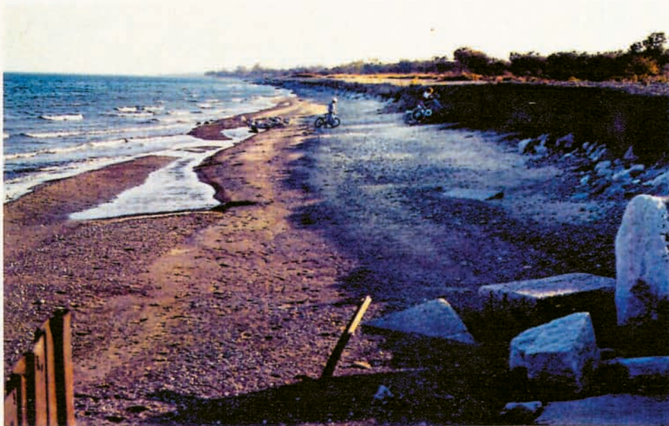
Figure 2-32 Same view as Figure 2-31 showing what remained of the South Unit nourishment stockpile in November 1995. The scarp crest has receded approximately 35 ft compared to the photo in Figure 2-31 to re-expose the riprap that defends this reach of shore (Photo date November 8, 1995).
