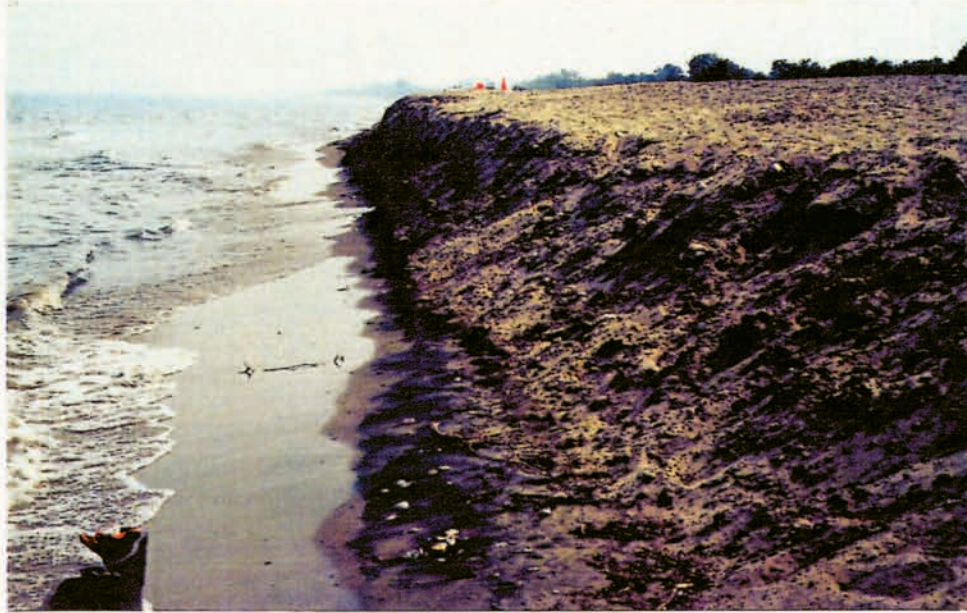
Figure 2-31 View looking southward along the South Unit nourishment site three days before completion of the June/July 1995 nourishment. Photograph is taken from the steel sheetpile (lower left) that defends the north end of the South Unit shoreline. Approximately 10 ft of recession has already occurred (Photo date July 11, 1995).
