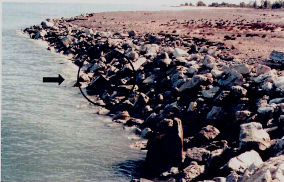
Figure 2-16 View of the riprap looking south from the south breakwater in October 1989. Note the variety of stone sizes and shapes. For comparison with the photograph in Figure 2-17, note the position and height above water of the concrete block supporting an upright steel pole, at left center with black arrow (Photo date October 4, 1989).
