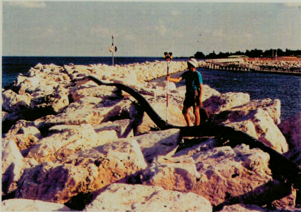
Figure 2-22 View showing localized subsidence of capstones along the middle section of the south breakwater. Discharge pipe for hydraulic dredging lies along the breakwater crest. This sag is located about 360 ft north of the inner daymarker which is visible in the distance. Note colored 1-ft increment bands on the prism pole for scale (Photo date July 18, 1995).
