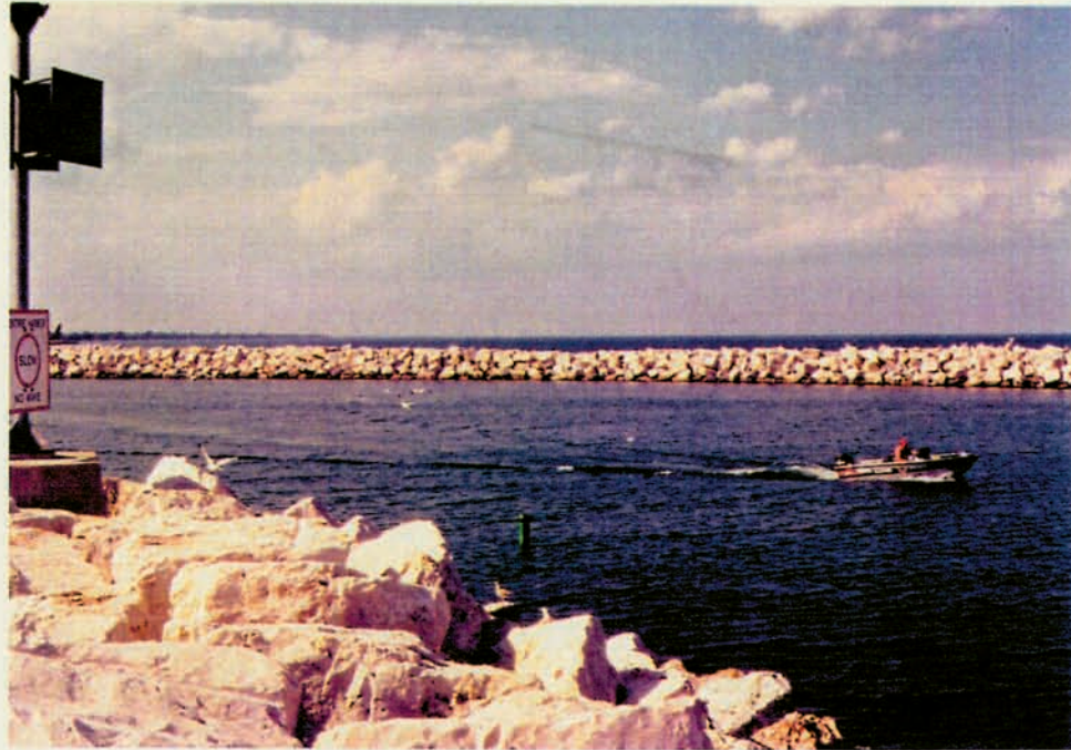
Figure 2-21A View looking north toward the north breakwater "sag" from the north end of the south breakwater. The extent of a sag in the crest can be seen by comparing the breakwater crest against the horizon. The sag is located between the inner and outer daymarkers (not visible in the photo) (Photo date July 18, 1995).
