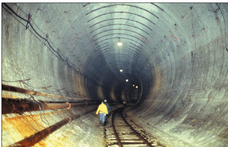
A person provides scale within an unlined tunnel segment in Silurian dolomite. This photo is from a tunnel system similar to TARP being built in Milwaukee County, Wisconsin (photo by Robert Bauer, ISGS).
