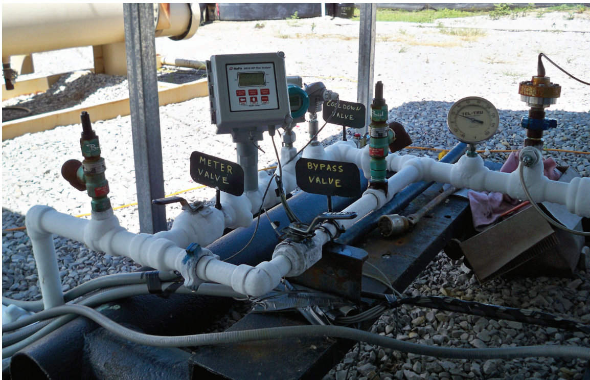
Figure 55 Cameron NuFlo liquid turbine meter (center, immediately behind "meter valve" sign) and Siemens pressure gauge (with blue cover, immediately behind NuFlo meter) in series on frosted line. In-line heater in upper left background. Tel-Tru mechanical temperature gauge at right is connected to pump discharge line. Photo courtesy of Trimeric Corp.
