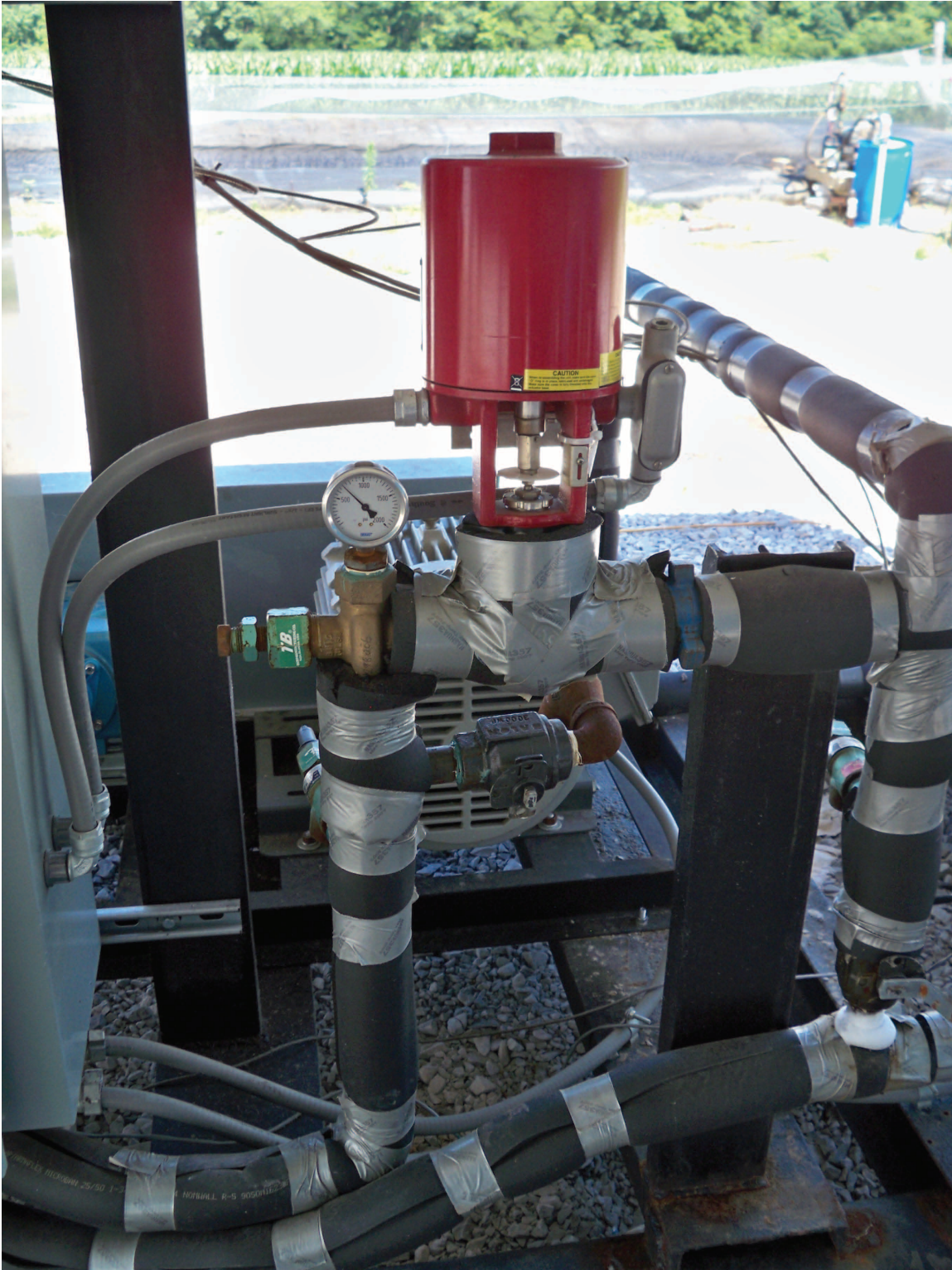
Figure 52 Globe Cast (BadgerMeter, Inc.) pressure control valve (red object at upper center) on return line between discharge of main pump and storage tank. The red casing conceals an electric actuator. The valve is below the actuator and is covered with black neoprene and gray duct tape. Photo courtesy of Trimeric Corp.
