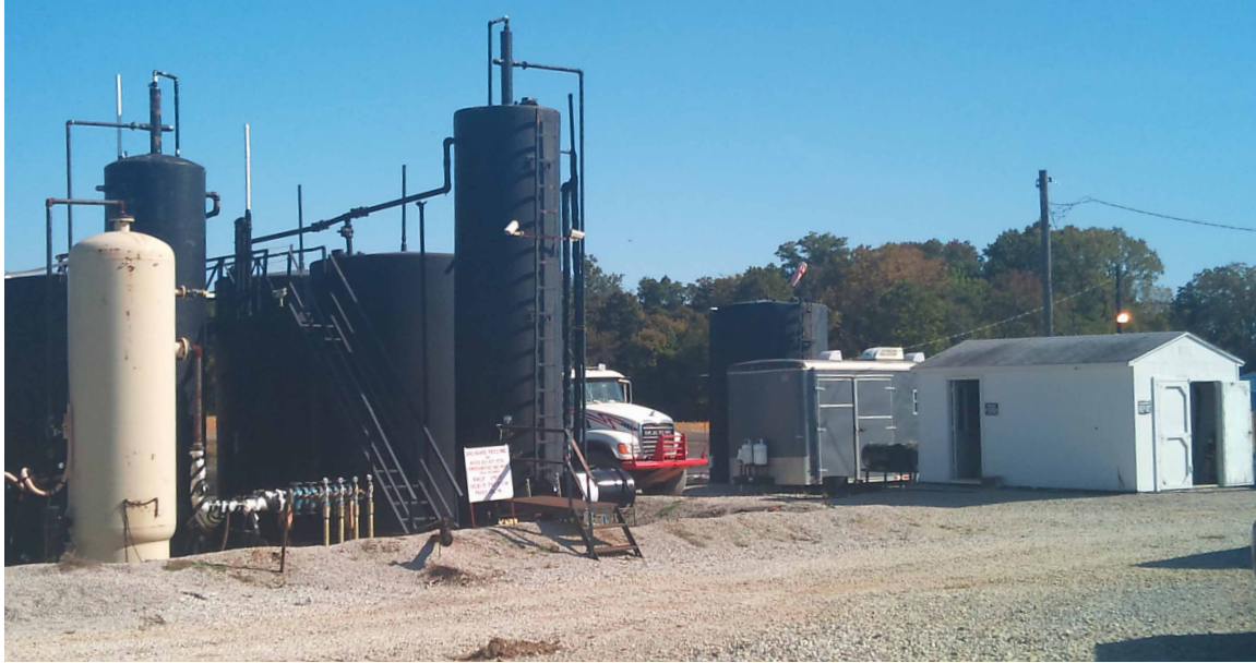
Figure 4 The tank battery at Mumford Hills Field, including tanks and pump house. Tanks are to the left, and the water injection equipment and accessories are in the white pump house at right.
