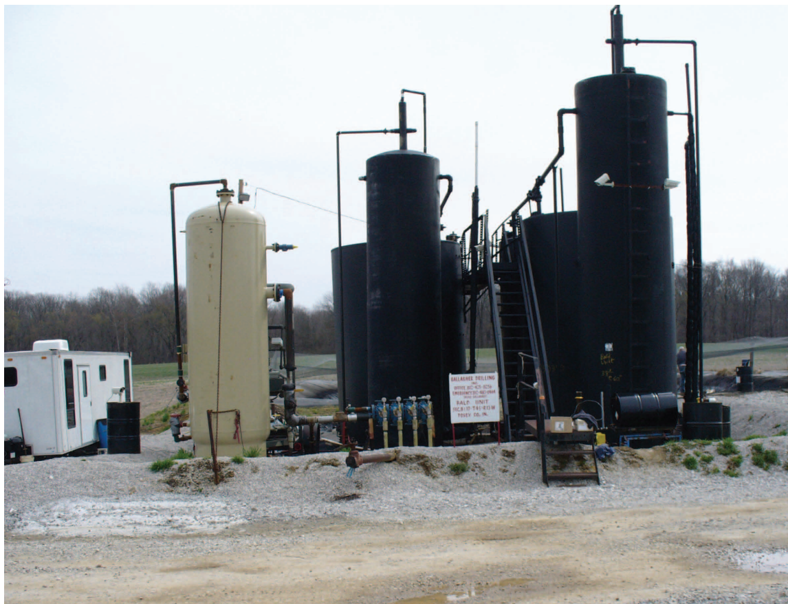
Figure 14 Bald Unit tank battery. The light-colored tank at left is the gas-liquid separator. The taller black tank behind the production manifold is the Natco “gun barrel” oil-water separator. The shorter black tanks behind the gun barrel are oil tanks. The second gun barrel at right was not used in the pilot project; BU-4 production was isolated from the pilot production and was sent to this gun barrel and to separate oil tanks.
