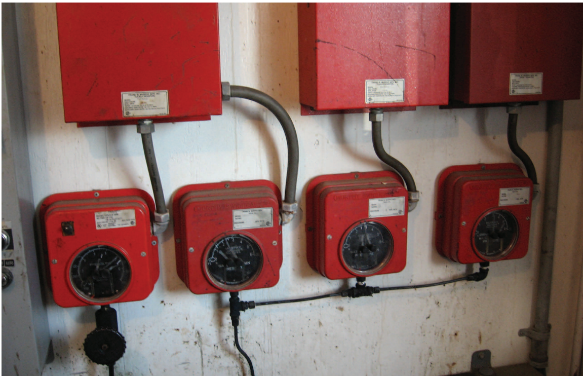
Figure 15 Example of control panels for water injection equipment in the Bald Unit pump house. (The photograph is from Sugar Creek Field.)
