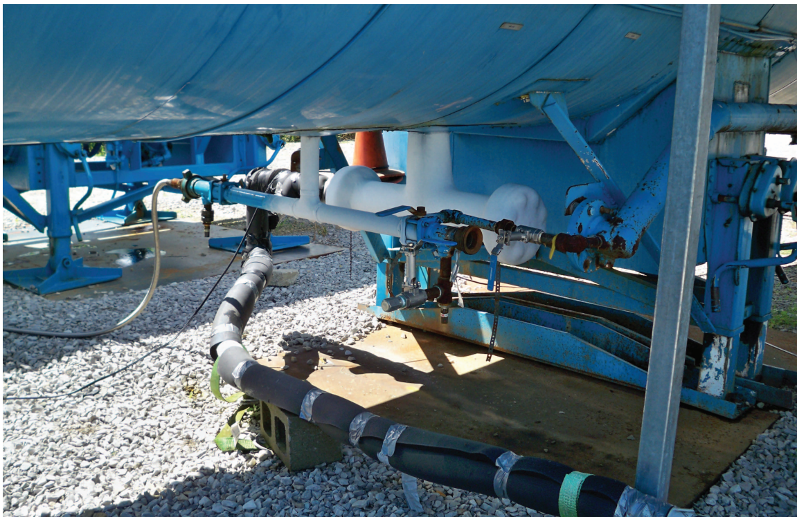
Figure 47 Connection line between CO 2 storage tank and injection equipment. Photo courtesy of Trimeric Corp.
