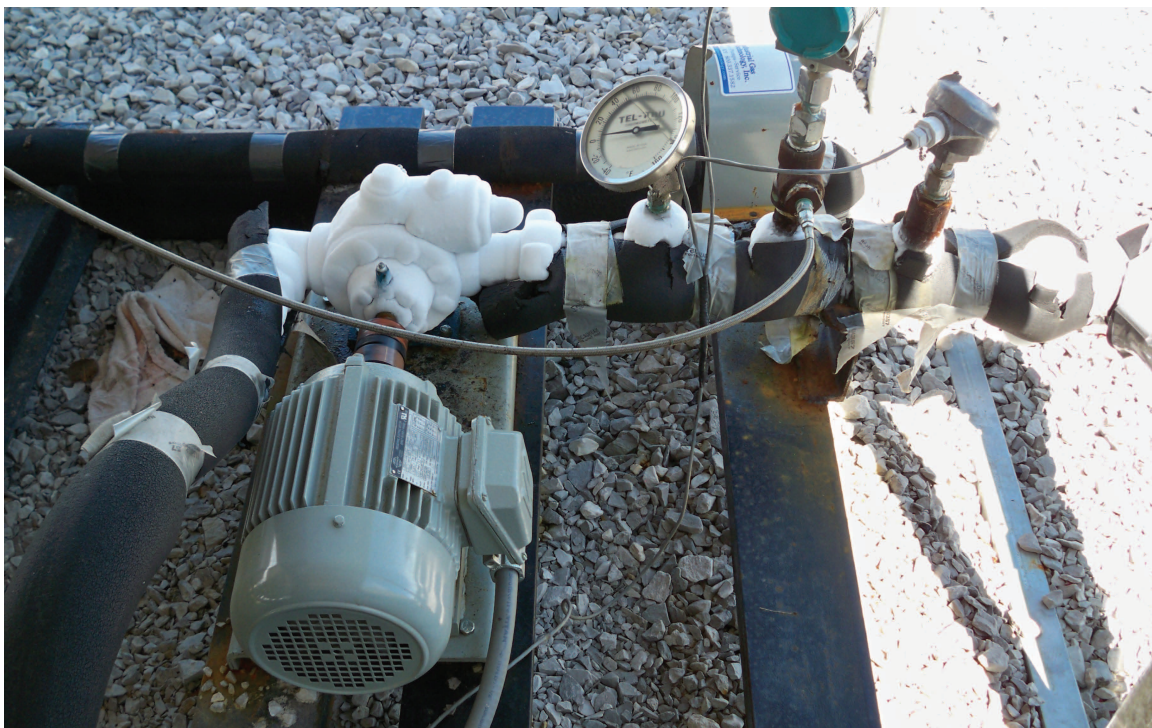
Figure 48 Booster pump (frosted over) and motor. The circular dial at the upper center of the photo (labeled Tel-Tru) is a manual temperature gauge. A Siemens pressure gauge (green-blue back, partially out of frame at upper right of photo) is located to the right of the manual gauge. Lines are covered with neoprene pipe insulation. The storage tanks are to the right; the main pump is to the left. Photo courtesy of Trimeric Corp.
