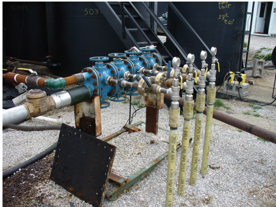
Figure 13 Production manifold at Bald Unit tank battery. Four vertical production flow pipes are in the foreground at center. Mani-Flo dual valve flow diverters are painted blue. Baker chokes (brass with blue handle) are between the flow diverters and the stainless-steel tees. The tees are topped with mechanical pressure gauges (backs shown). The large gray line to left leads to the gas-liquid separator.
