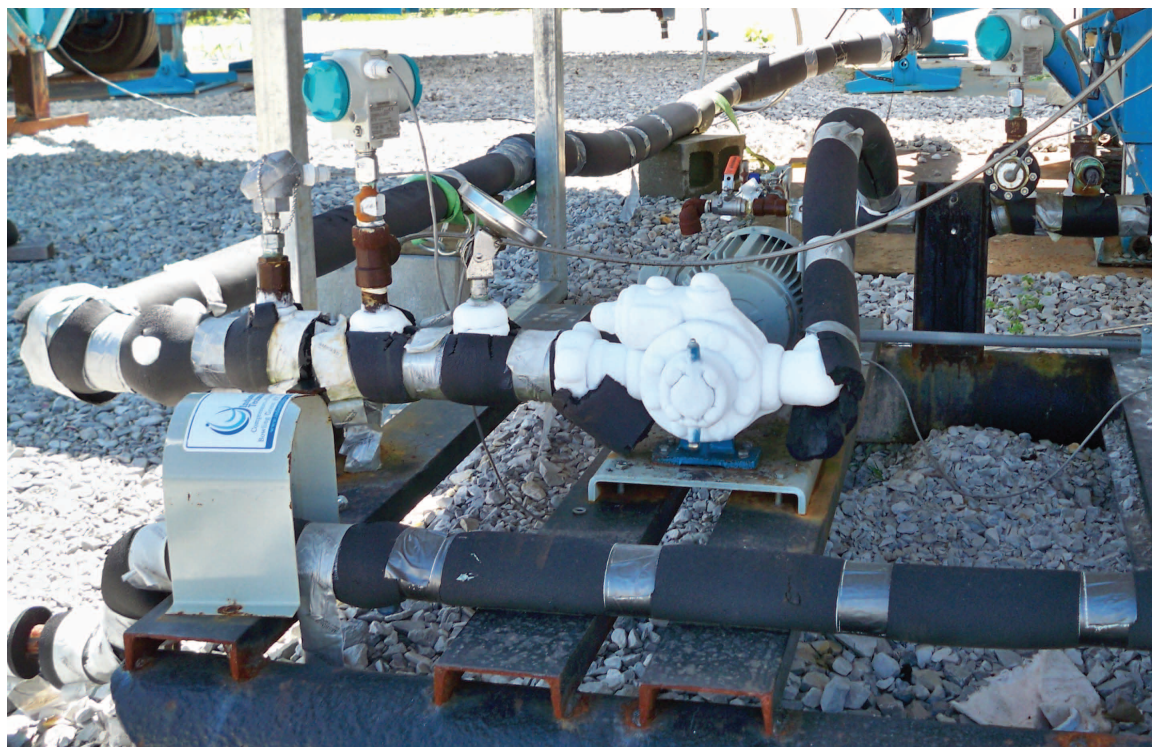
Figure 49 Injection pump skid at the Bald Unit tank battery. Frosted-over booster pump and motor seen in Figure 48 are visible at center. CO 2 tank supports are visible in background. Photo courtesy of Trimeric Corp.
