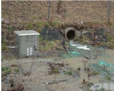
7d. TB9Ac2N 1.5-ft culvert
