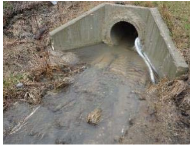
7b. TB7Bout 2-ft culvert
