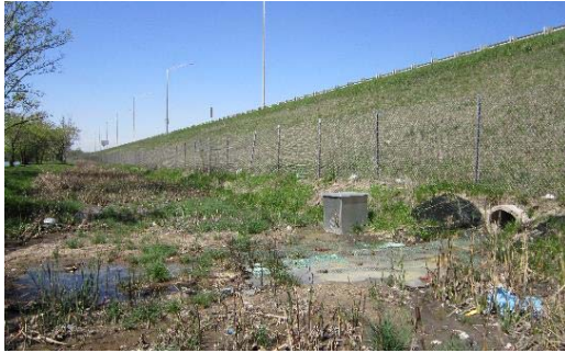
4b. Post-construction outlet TB9A, view to south
