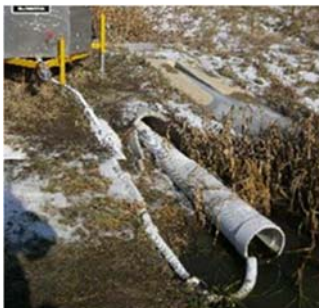
7g. TB15Bgw 8-in. underdrain pipe
