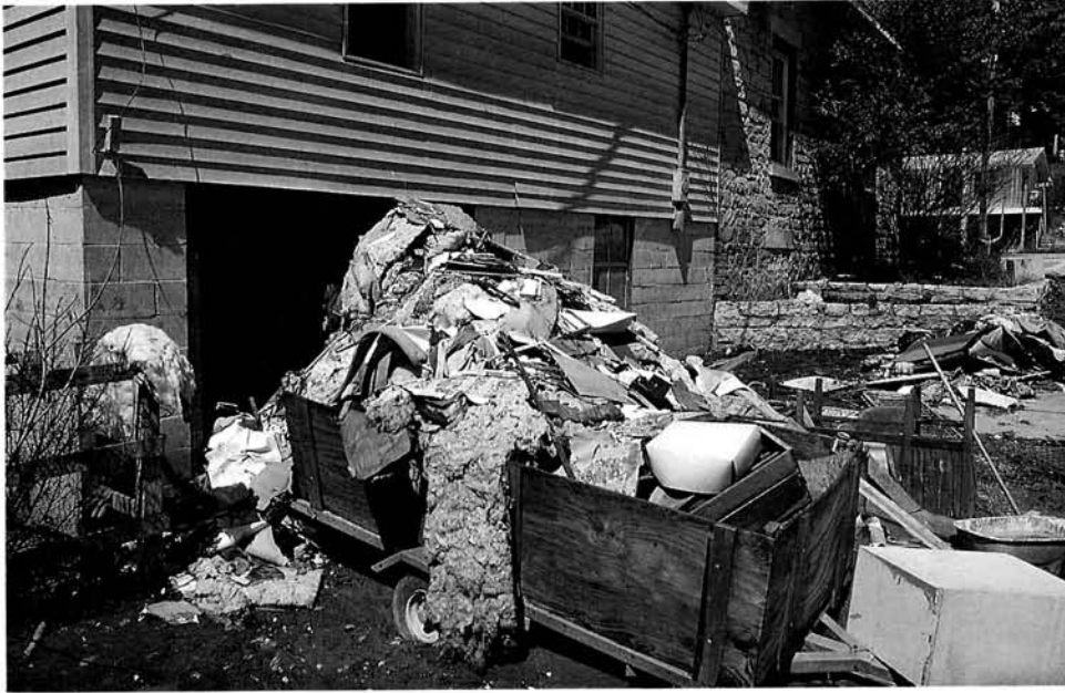
5 Jersey County: Aerial view (below) shows how much of Grafton was flooded at about the time of the highest flood crest (August 6, 1993). Water-saturated plasterboard and insulation removed from flood-damaged houses such as this Grafton home (left) cannot be reused. The debris from buildings affected by flood water will be a new burden on landfills. (September 3, 1993)
