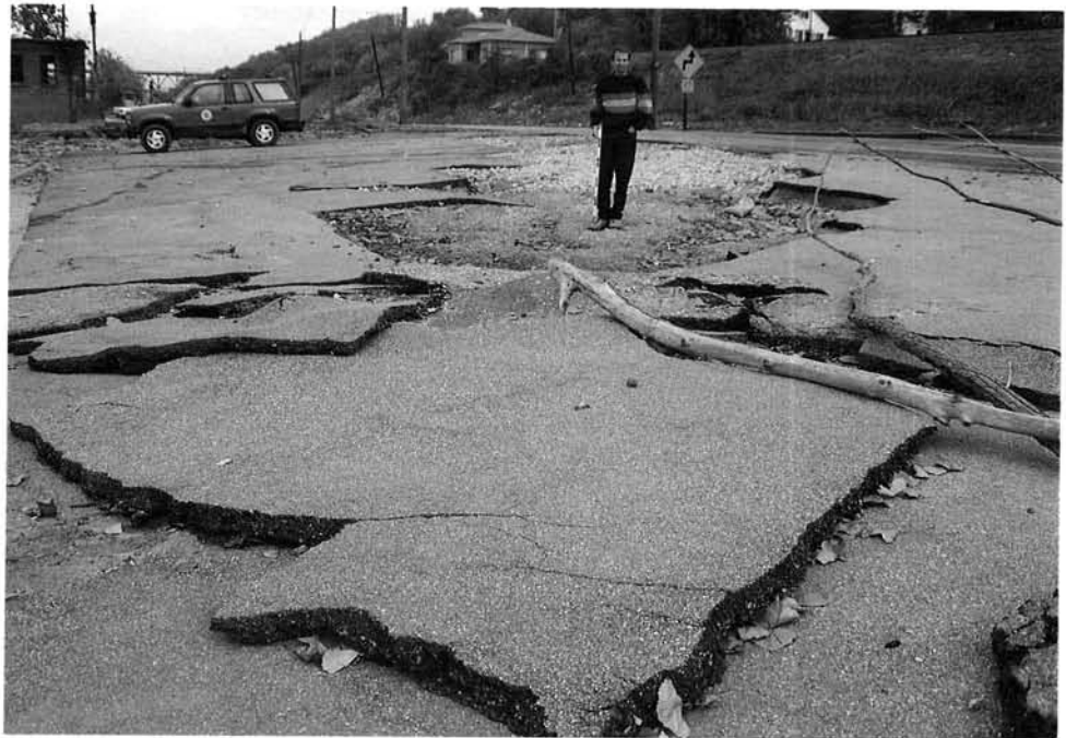
4 Randolph County: Asphalt pavement slabs next to the river-front road at Chester were lifted and transported by flood water. Robert Bauer, ISGS engineering geologist, stands where the blacktop slabs were eroded (October 13, 1993).
