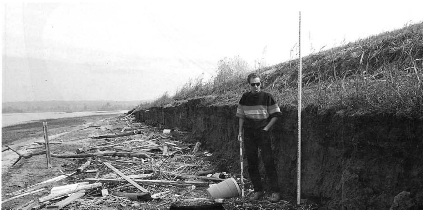
28 Randolph County: Nearly vertical cut made by waves eroding the inner (landward) side of the southern part of the Kaskaskia Island levee. Note the driftwood and debris where ISGS engineering geologist, Robert Bauer, stands at the base of the erosional cut (October 13, 1993).
